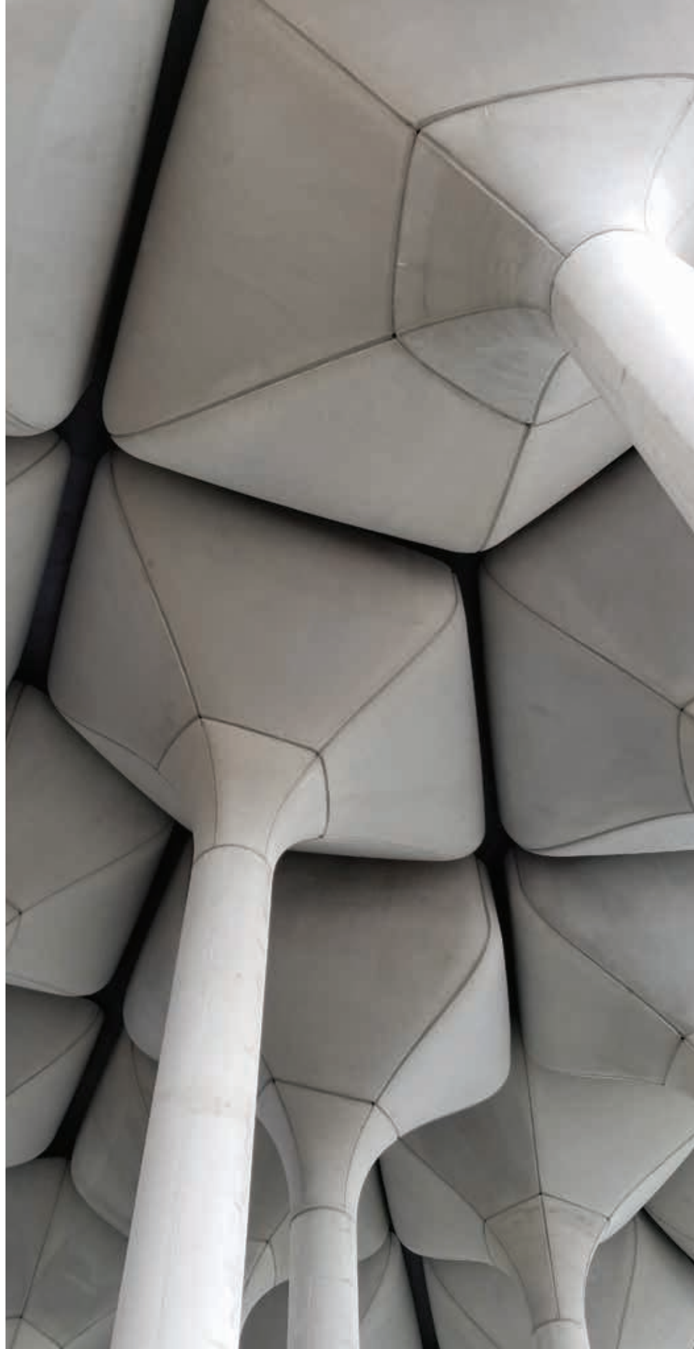
The underside of some of the 132 pots installed at Little Island.
