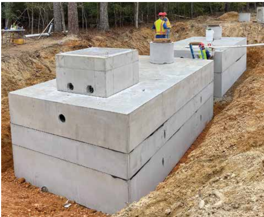
Each tank consisted of three sections, with the top and bottom sections weighing 21,000 pounds a piece and the middle 14,000 pounds.
