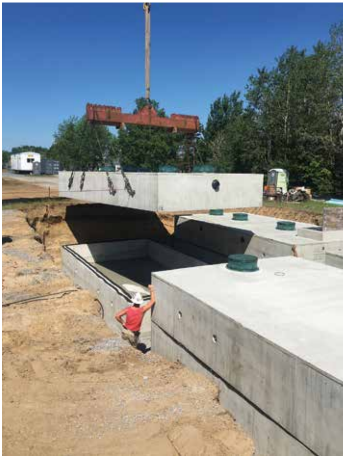
The tanks installed for the Brushton-Moira schools were set in one day.
