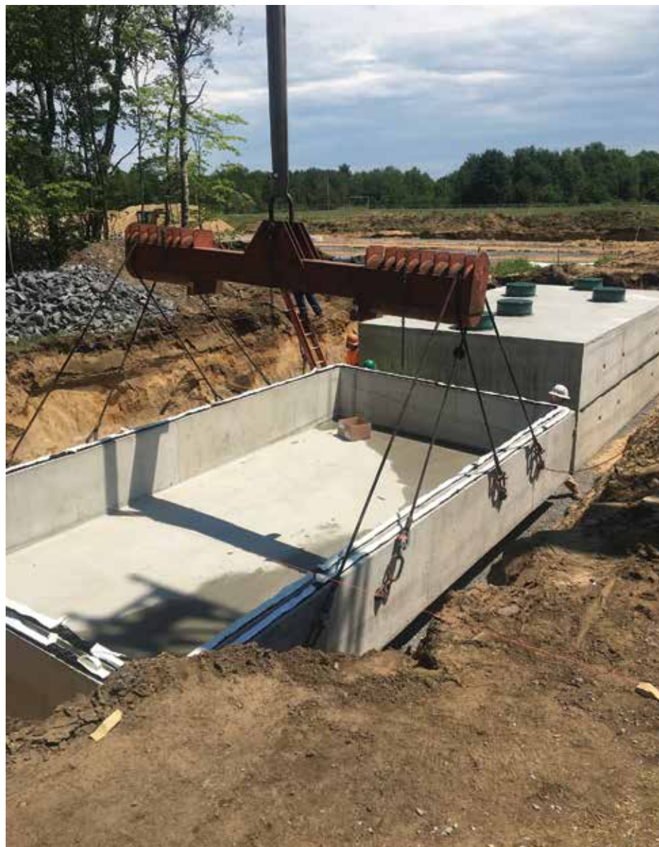
Camp Precast provided four 10,000-gallon septic tanks for the Brushton-Moira Central School District.
