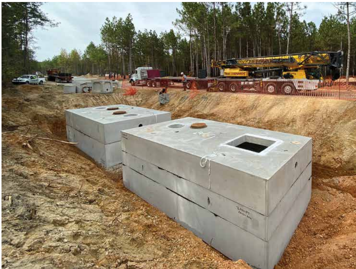
Shoaf Precast manufactured the precast portions of the septic system for the Moccasin Branch campground at Raven Rock State Park in North Carolina.
