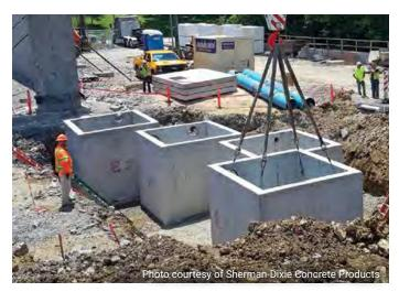
A series of precast concrete cisterns is installed for a fire department in Green Hills, Tenn.
