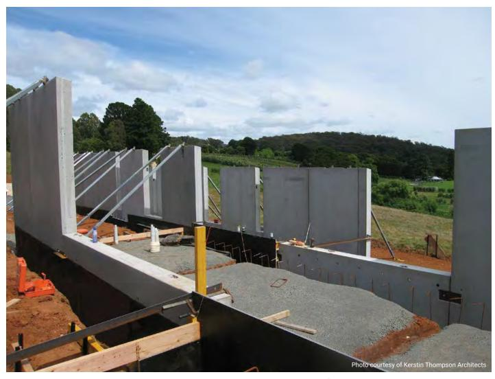
Thermal insulated concrete sandwich panels keep the home's temperature consistent despite extreme fluctuations in the area.
