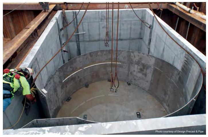
Each of the 14 large precast stormwater structures contains a vortex swirl chamber that removes waste, oil and sediments from the captured water.
