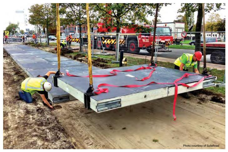
Construction workers install precast concrete solar panels for the 230-foot-long SolaRoad bike path in the Netherlands.
