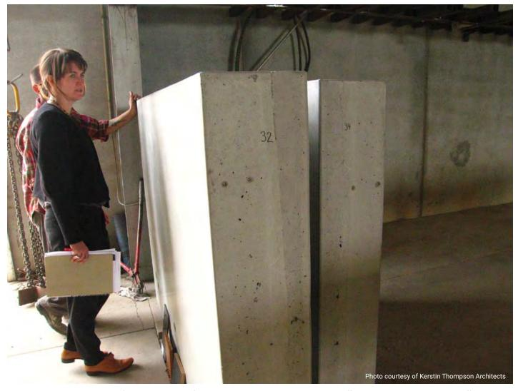
Kerstin Thompson Architects specified precast concrete for the House at Hanging Rock due to its cost-effectiveness, durability and thermal efficiencies.
