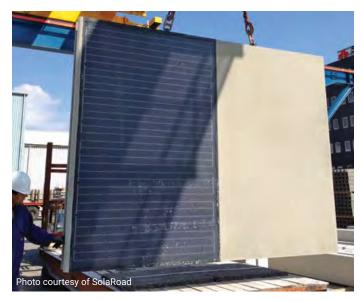
The SolaRoad bike path in the Netherlands consists of precast concrete panels with a translucent top layer of tempered glass.
