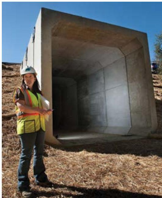
It is popular where there are environmental issues or a desire to avoid disturbance to a stream bed. This structure can sit on a CIP footing situated on opposite sides of a stream. The three-sided arch spans the stream without adversely affecting the stream's natural state.
