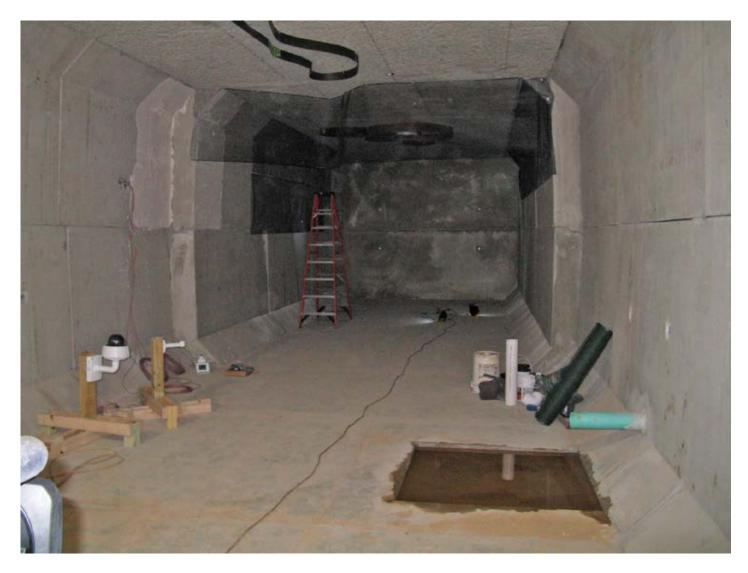
The Nature Conservancy in Tennessee used a modified box culvert from Oldcastle Precast in Lebanon, Tenn., to create an artificial bat cave as part of its efforts to save the Little Brown Bat from a population-devastating fungus. n the 1980s, Transformers<sup>i</sup> burst on the scene as a must-have toy thanks to some ingenuity and creativity. They are, after all, "more than meets the eye."
