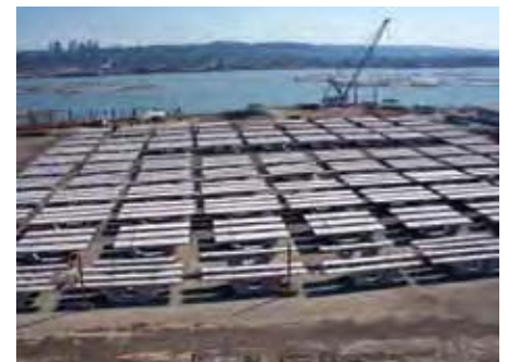
BRIDGE SEGMENTS FOR THE PORT MANN BRIDGE
