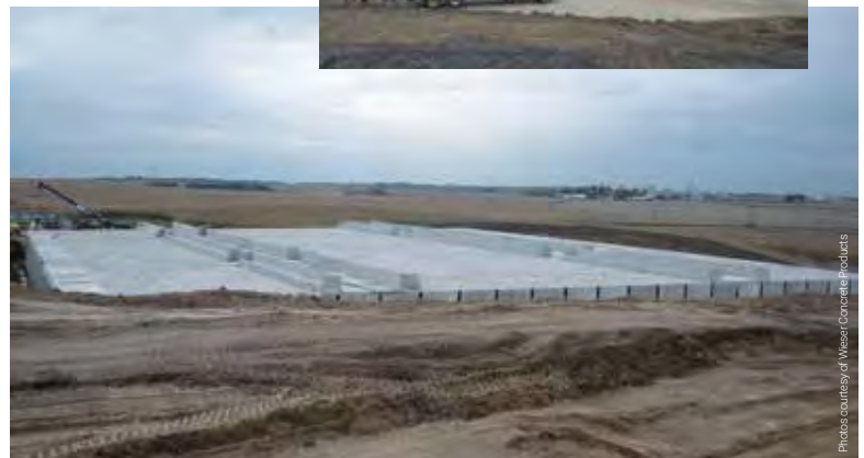
Slatted-Floor Under-Barn Manure Storage System
