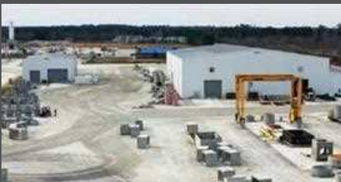
TOP TO BOTTOM: BUD KNIGHT BUILT HIS FIRST PUMPER TRUCK TO START HIS BUSINESS; BUD KNIGHT'S FIRST BUILDING, WHERE HE BEGAN POURING SEPTIC TANKS; EXPANSION OF THE SECOND PLANT PROVIDED MORE SQUARE FOOTAGE AND ADDITIONAL HEIGHT; KNIGHT'S BATCH PLANT AND SEPTIC TANK BUILDING CAN BE SEEN IN THE BACKGROUND BEHIND ITS OFFICE AND TWO PRECAST BUILDINGS.
