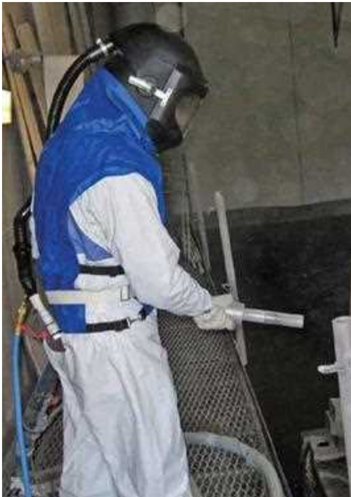
NON-SILICA (SAND) ABRASIVES MAY STILL GENERATE SILICA DUST WHEN ABRASIVE-BLASTING CONCRETE PRODUCTS. NIOSH-CERTIFIED SUPPLIED-AIR ABRASIVE BLAST HELMETS MUST BE USED. Photo courtesy of 3M
