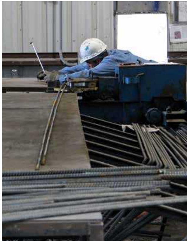
Employees take care of all aspects of production, including bending and cutting rebar.
