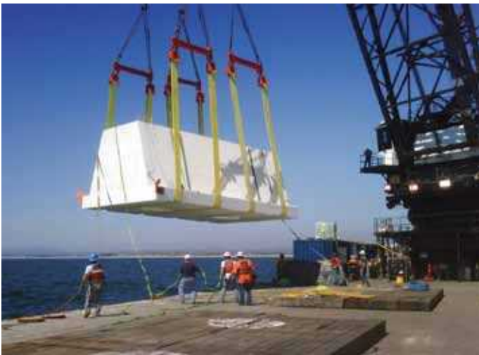
U.S. CONCRETE PRECAST GROUP - SOUTHERN CALIFORNIA – MAGNETOMETER STABILIZATION CAISSONS
