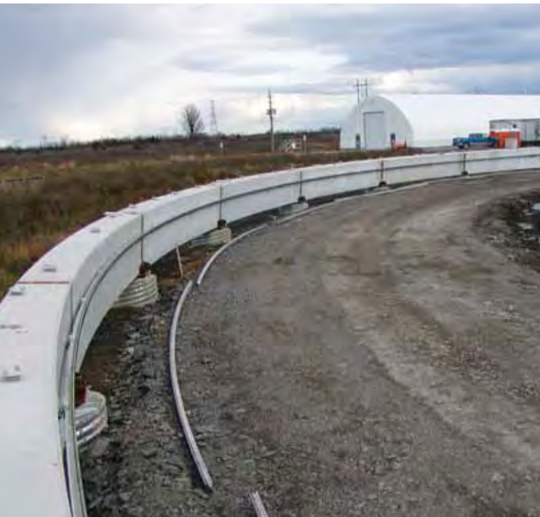
ANCHOR CONCRETE PRODUCTS – MONORAIL TEST TRACK FOR BOMBARDIER TRANSPORTATION SYSTEMS
