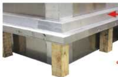
Pallet Forms placed on Riser Forms.
