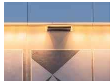
The abstract flower pattern, designed by Spanish-born artist Dani Marti, spans across 30 precast concrete panels, each nearly 40 feet high.
