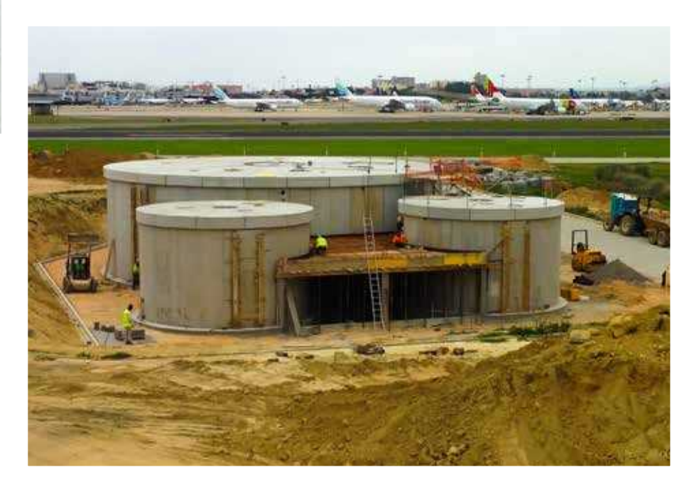
The largest of the three precast concrete water tanks manufactured for the Lisbon Airport in Portugal holds about 450,000 gallons of water.
