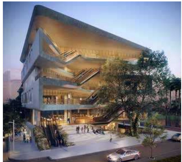
Banyan trees provided design inspiration for the custom branching pattern stamped on the exposed precast concrete.
