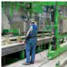
Wall production line
