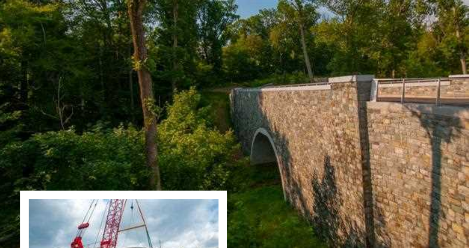
Above: Faddis manufactured a twin leaf, 42-foot-span arch in the new Millenium project section of Arlington National Cemetery.
