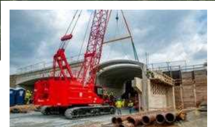
Above: Faddis manufactured a twin leaf, 42-foot-span arch in the new Millenium project section of Arlington National Cemetery.
