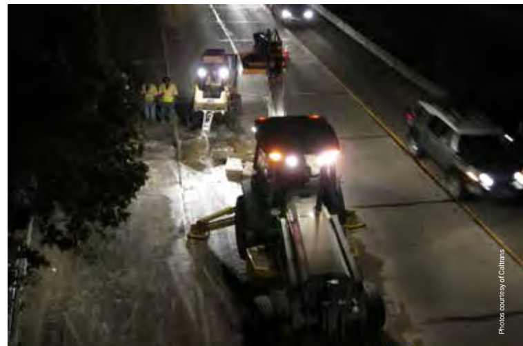
Precast concrete pavement panels allow for rapid repair and construction.
