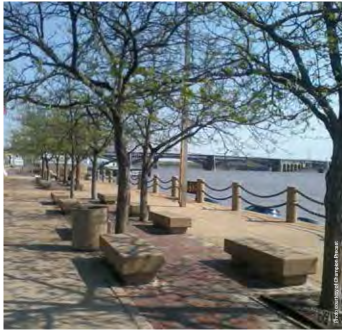
Precast concrete bollards obstruct vehicular traffic and protect pedestrians in St. Louis, Mo.
