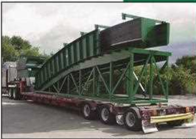
ARCHED BRIDGE BEAM
