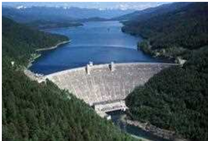
THE HUNGRY HORSE DAM, STARTED IN 1948 AND COMPLETED IN 1953, MARKED THE FIRST SIGNIFICANT USE OF FLY ASH IN CONCRETE. Photo courtesy of U.S. Bureau of Land Management
