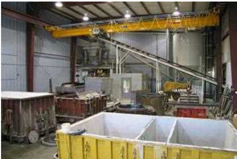
PLANT MODERNIZATION AT DALMARAY CONCRETE PRODUCTS INC., JANESVILLE, WIS.
