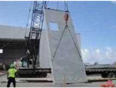
A U.S. COAST GUARD HANGAR, FEATURING ALL-PRECAST CONSTRUCTION INCLUDING ITS DOORS, TAKES SHAPE IN THE BAHAMAS.
