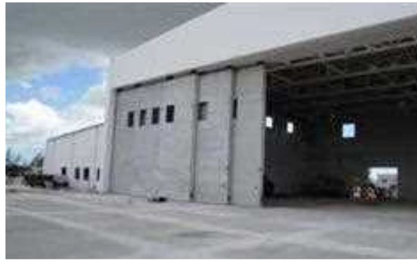
A U.S. COAST GUARD HANGAR, FEATURING ALL-PRECAST CONSTRUCTION INCLUDING ITS DOORS, TAKES SHAPE IN THE BAHAMAS.
