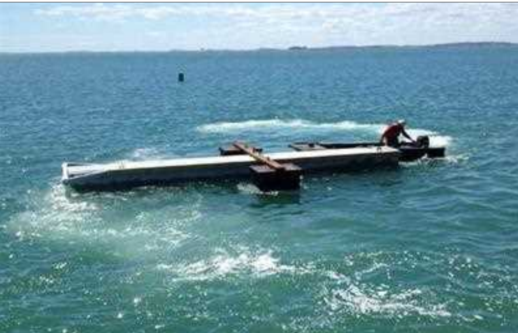
AFTER ARRIVAL ON SITE, MANY OF THE DOCKS HAD TO BE FLOATED BY TUGBOATS TO THEIR DESTINATIONS, WHERE THEY WERE LIFTED AND LOWERED INTO PLACE. Photos courtesy of Shea Concrete Products
