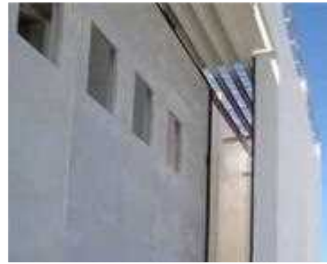
A U.S. COAST GUARD HANGAR, FEATURING ALL-PRECAST CONSTRUCTION INCLUDING ITS DOORS, TAKES SHAPE IN THE BAHAMAS.
