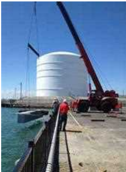
AFTER ARRIVAL ON SITE, MANY OF THE DOCKS HAD TO BE FLOATED BY TUGBOATS TO THEIR DESTINATIONS, WHERE THEY WERE LIFTED AND LOWERED INTO PLACE. Photos courtesy of Shea Concrete Products
