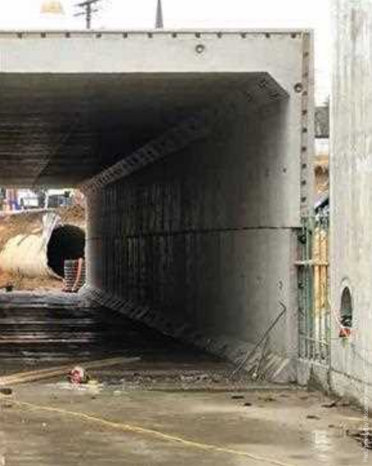
The new precast concrete culvert installed at Ellicott Mills Drive weighs 23 tons and is 140 feet long, 24 feet wide and 13 feet high.
