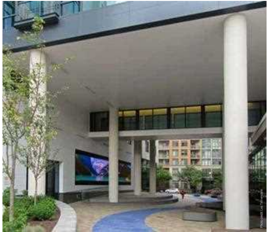
The high-thermal mass precast concrete wall panels absorb heat during the day, and then slowly release heat as temperatures drop at night.
