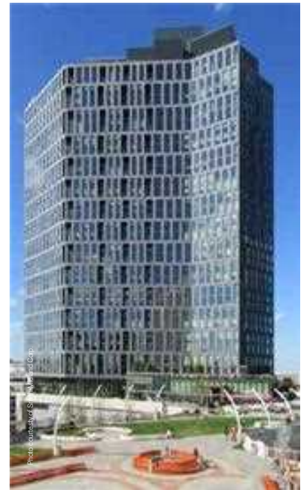
The VITA building in Tysons employs precast concrete panels with a unique shape and color to create a shape that implies a weave, like fabric.
