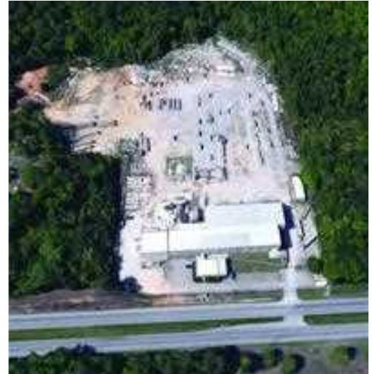
Aerial view of Smith-Columbia's 39-acre precast production facility in Hopkins, S.C.
