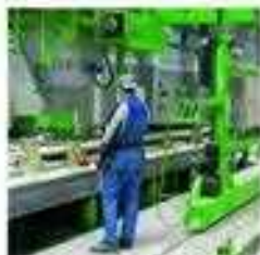
Wall production line
