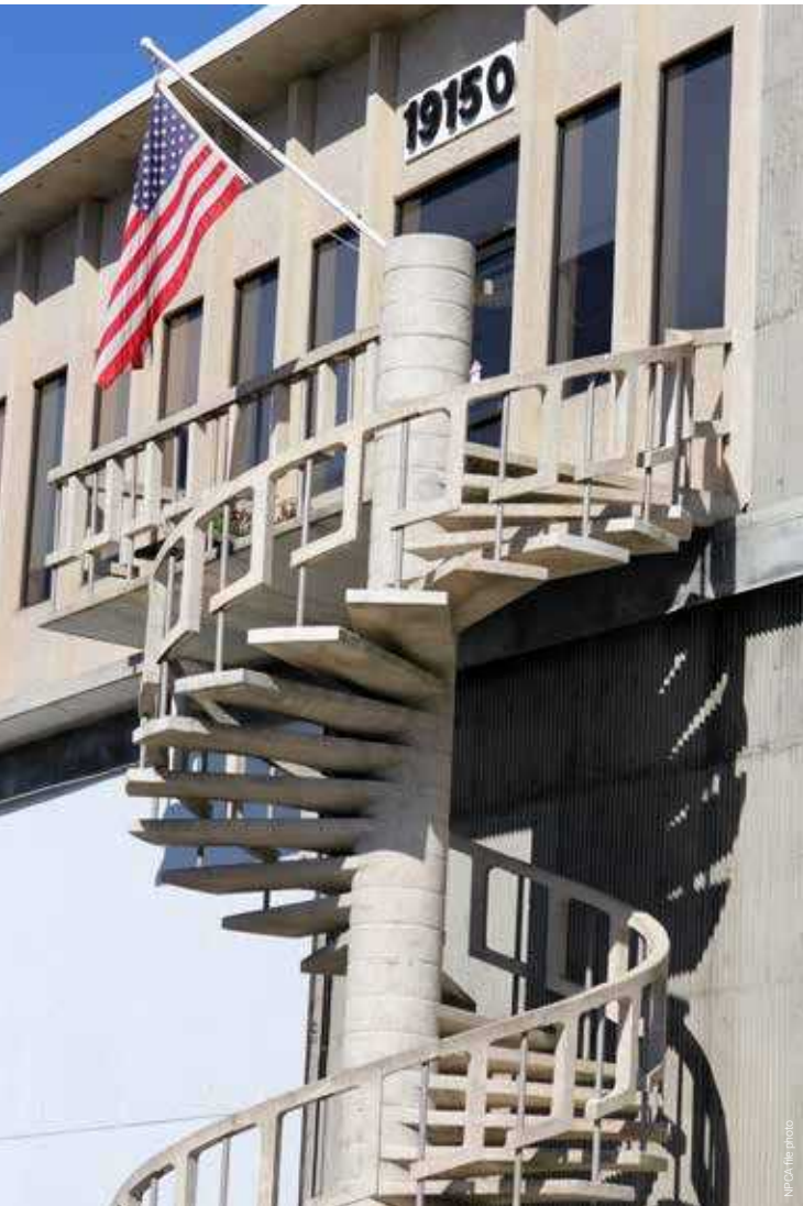
(Above) The original precast concrete building and cast stone spiral staircase built by Clarke Jewell's maternal grandfather, Ralph Robinson, continue to hold value and family traditions for the staff and leadership at Olympian Precast.
