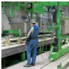
Wall production line
