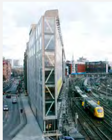
PRECAST PANELS WITH WINDOWS PREINSTALLED ELIMINATED THE NEED FOR SCAFFOLDING DURING CONSTRUCTION OF THE FLAT IRON BUILDING IN STOCKHOLM, SWEDEN. Photo courtesy of Skanska AB
