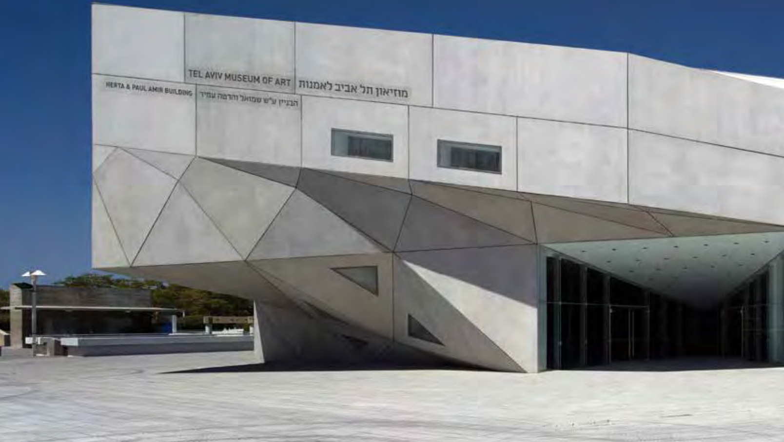
A RECENT EXPANSION TO THE TEL AVIV MUSEUM OF ART IN TEL AVIV, ISRAEL, INCLUDES AN EXTERIOR SHELL MADE OF 460 PRECAST CONCRETE PANELS. Photo courtesy of Preston Scott Cohen Inc.
