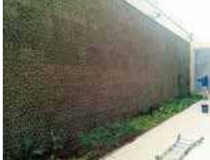
Besser's ECONcrete bioactive wall
