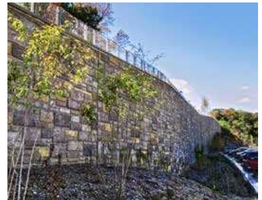
Smithsonian's National Zoological Park Retaining Wall by Smith-Midland
