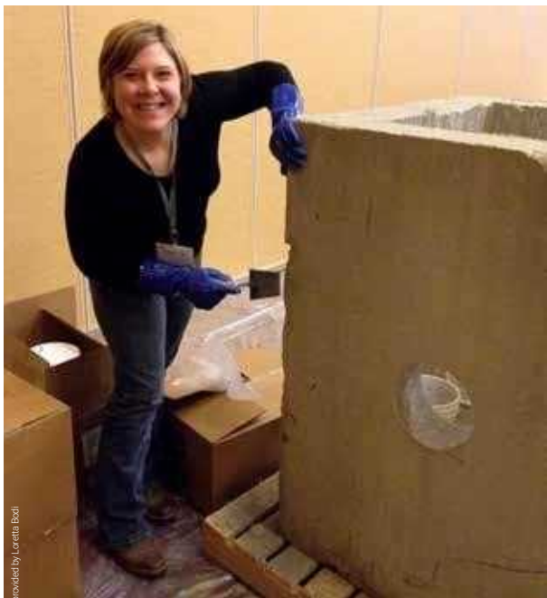
Loretta Bodi learned how to repair a catch basin in PQS II - Production.
