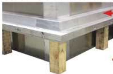
Pallet Forms placed on Riser Forms.
