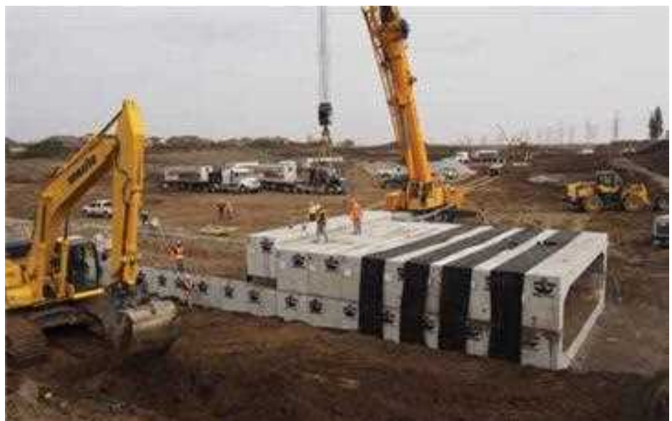
HIGHWAY 407 EAST EXPANSION – WHITBY, ONTARIO
