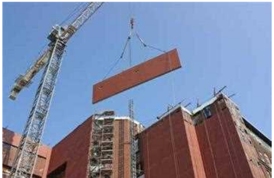
NELSON HARVEY FACILITY, JOHNS HOPKINS MEDICINE CAMPUS
