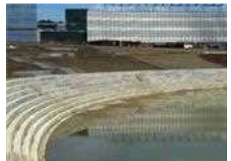
EATON CORPORATE HEADQUARTERS REFLECTING POND WALL
