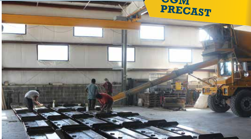
CGM'S NEW PRODUCTION BUILDING INCORPORATED HIGH SOUTH-FACING WINDOWS FOR NATURAL LIGHT.
