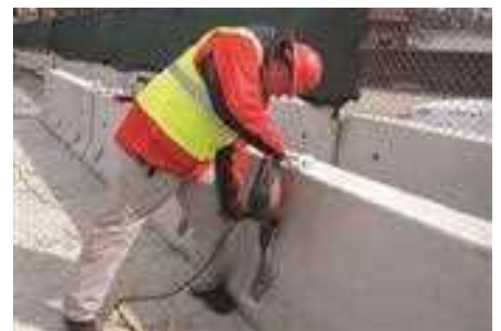
J-J HOOKS MASH TL3 BRIDGE INSTALLATION
