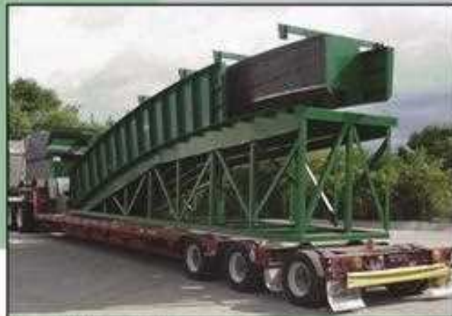
ARCHED BRIDGE BEAM
