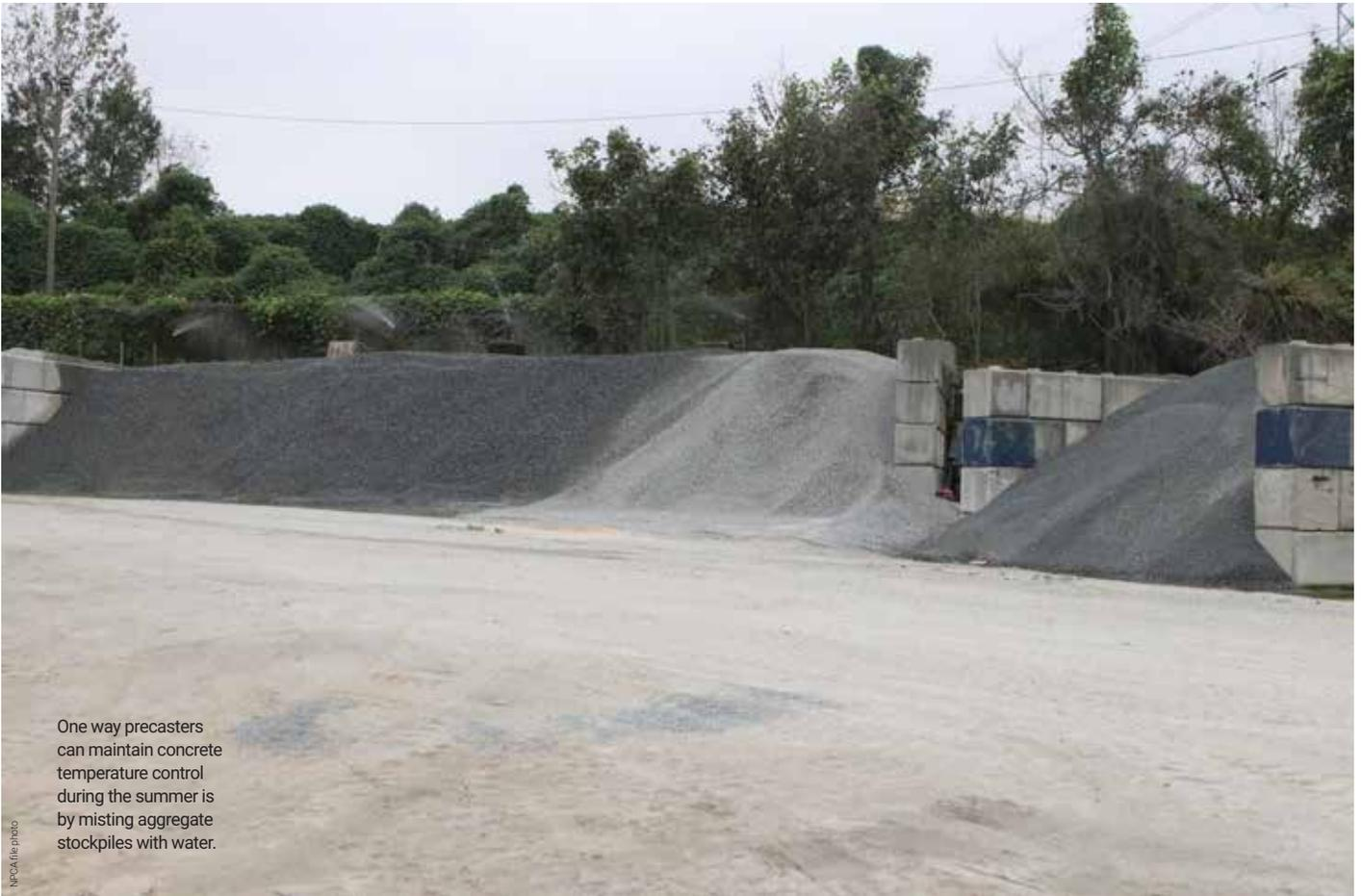
One way precasters can maintain concrete temperature control during the summer is by misting aggregate stockpiles with water.
