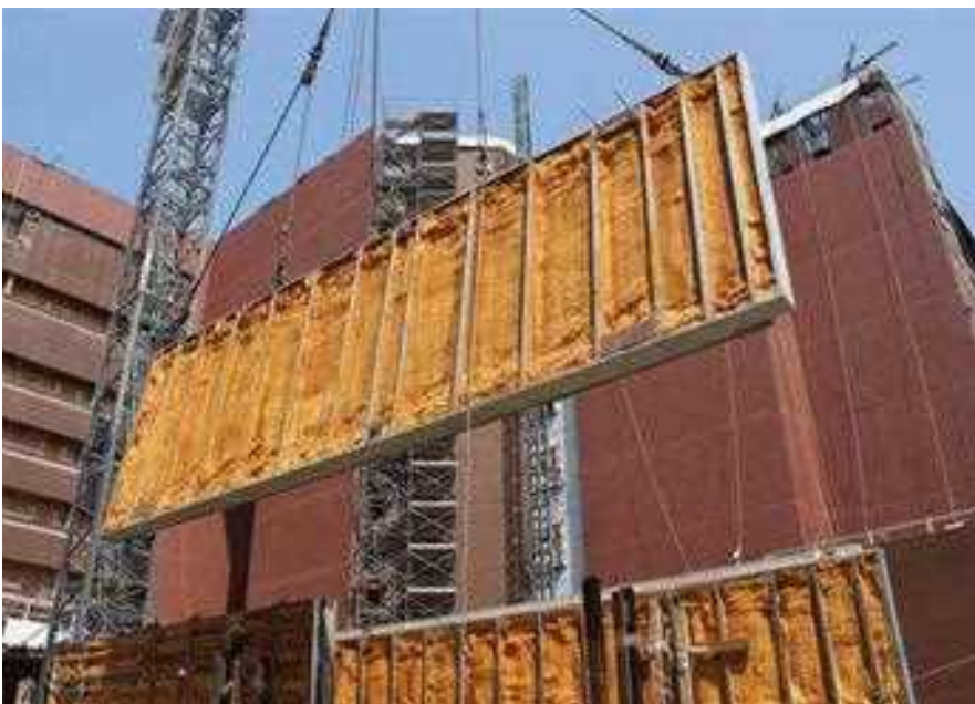
NELSON HARVEY FACILITY, JOHNS HOPKINS MEDICINE CAMPUS
