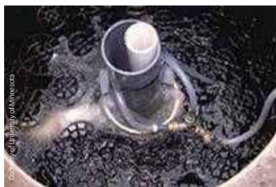
Aeration in an ATU breaks down organic matter.
