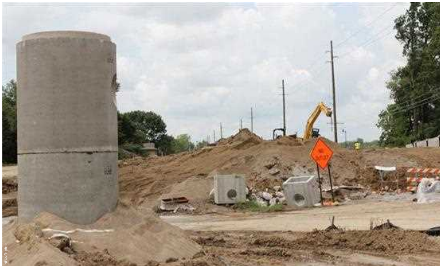
Precast circular manhole sections for drainage per AASHTO M199 (ASTM C478) positioned for DOT deep burial.
