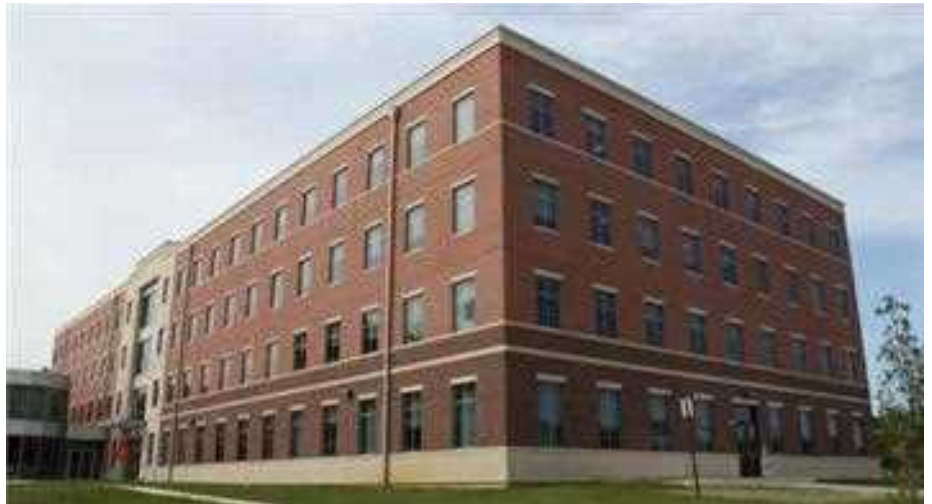
THE U.S. LEGAL SERVICES AGENCY ADMINISTRATION BRAC 132 BUILDING IN FT. BELVOIR, VA., WITH ITS BRICK-CLAD PRECAST CONCRETE WALL PANELS, IS A CERTIFIED LEED GOLD PROJECT. Photo courtesy of Smith-Midland Corp. ( smithmidland.com )
