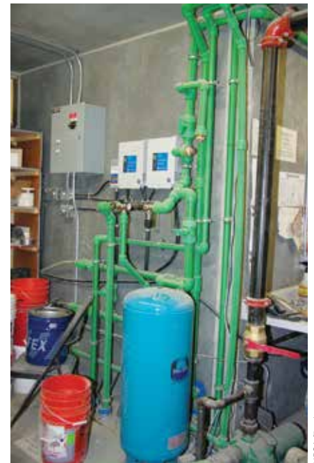
RATHER THAN DISCHARGING PROCESS WATER, PRODUCERS CAN TREAT IT WITH A RECYCLING SYSTEM.
