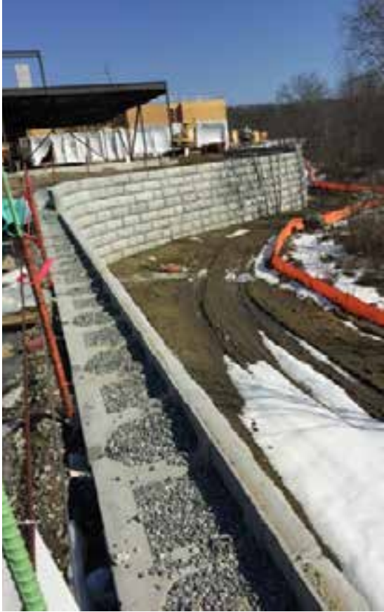
MBO manufactured a retaining wall for a sports complex in Massachusetts.
