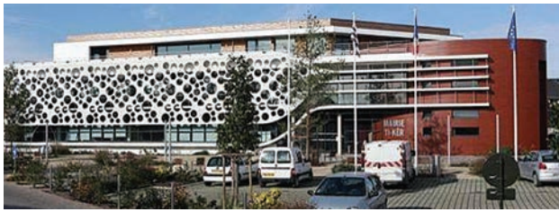
Figures 18, 19 – Perforated UHPC panels at Plescop City Hall, France (Photos courtesy of Lafarge)
