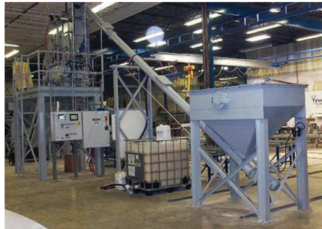
Figure 3 – UHPC batching facility (Photos courtesy of Lafarge)
