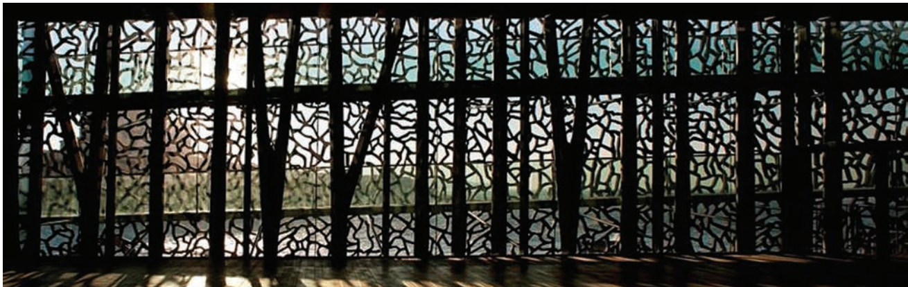
Figure 36 – MuCEM's UHPC lattice facade features tree-like, UHPC columns (Photo courtesy of Lisa Ricciotti)
