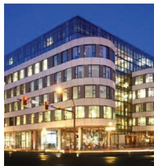
Figures 11, 12 – The Atrium, Victoria, B.C. features an ultra-thin, unitized curtain wall system.
