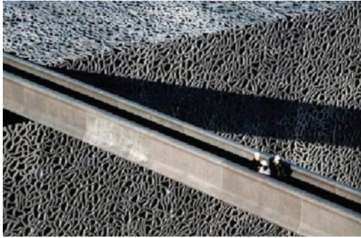
Figures 34, 35 – Mega project: MuCEM with UHPC lattice facade, roof and footbridge. (Photo courtesy of Lisa Ricciotti)
