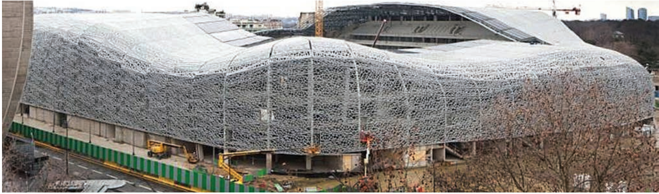
Figure 32 – Mega project: Stade Jean Bouin, a 23,000 square meter UHPC lattice envelope and roof (Photo: Nanick Guihodo)
