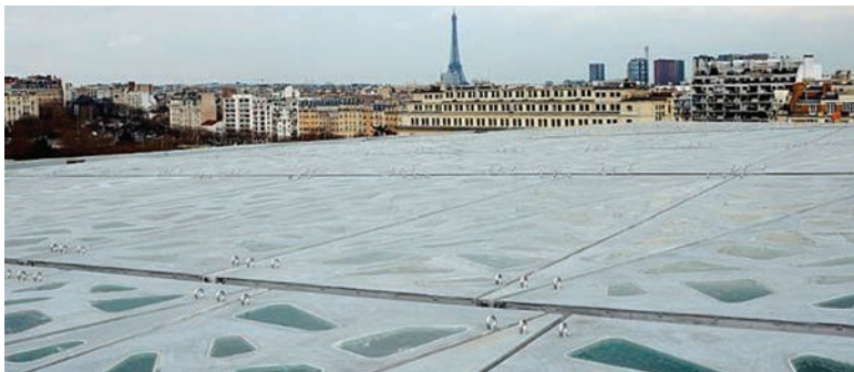
Figure 33 – (left) Stade Jean Bouin's UHPC lattice roof system with glass inserts (Photo courtesy of Olivier Amsellem); (right) the open lattice facade allows sunlight to filter through (Photo courtesy of Lisa Ricciotti)
