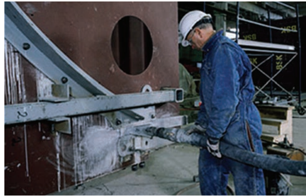
Figure 5 – Injection casting (Photo courtesy of Lafarge)
