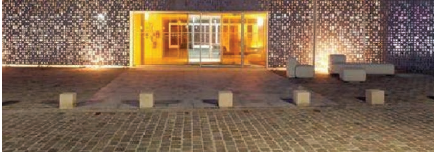
Figures 15, 16 – Community Center, Sedan, France perforated UHPC panels create a double-skin facade that provides privacy, sunshade and daylight.
