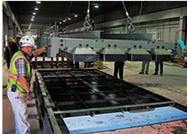
Figure 7 – Displacement casting (Photo courtesy of Lafarge)
