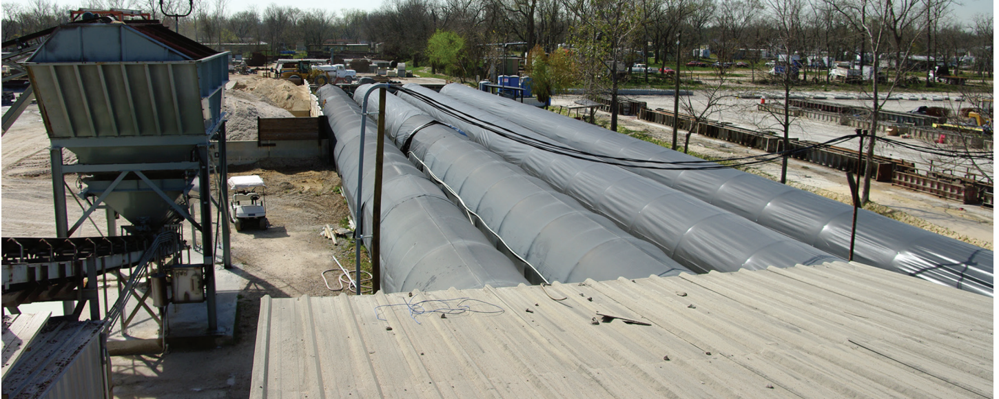
Curing enclosures used to maintain temperature and moisture
