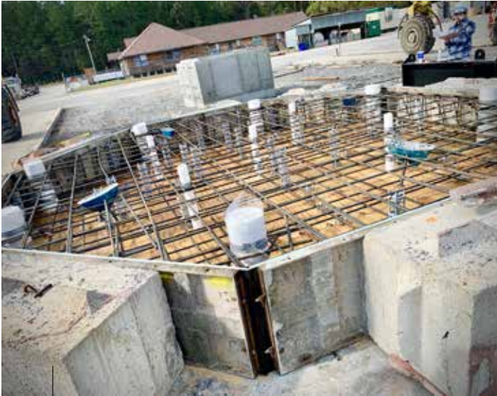
Left: A false floor is constructed inside the form to match the slope of the existing foundation underneath. Right: The completed slab with anti-slip surface finish is ready to be delivered and installed.
