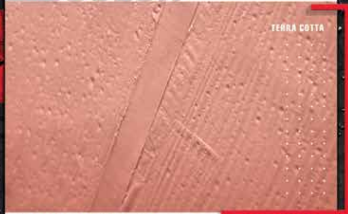
COLOR MATCHED WATERPROOF COATING & ELASTOMERIC JOINT SEALANT APPLIED TO ARCHITECTURAL CONCRETE JOINT
