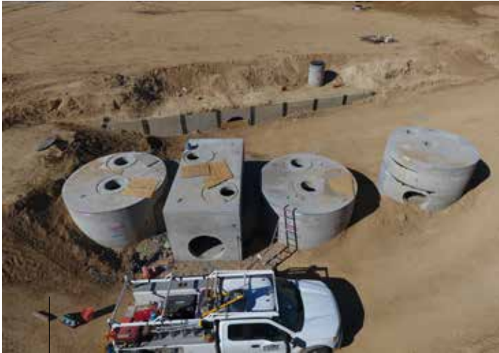
Corrugated metal pipe was originally specified for the project at Williams Ranch, but precast's durability made it the superior choice.
