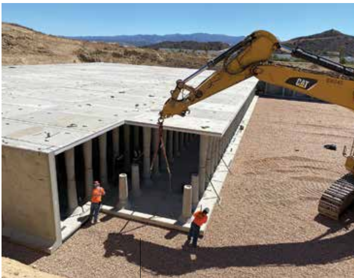
→ The open-air design allows for visibility for 300 feet diagonally throughout the system.
