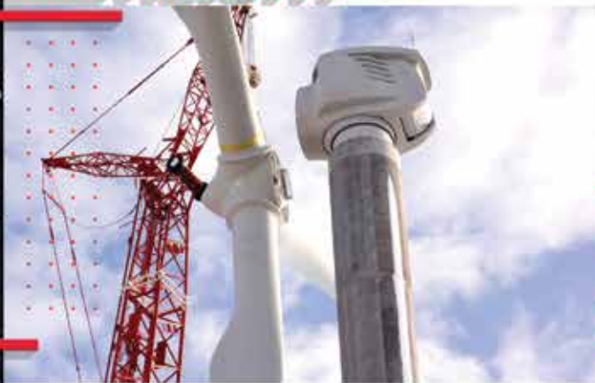
100 METER TALL (328 FEET) PRECAST WIND TURBINE TOWER
