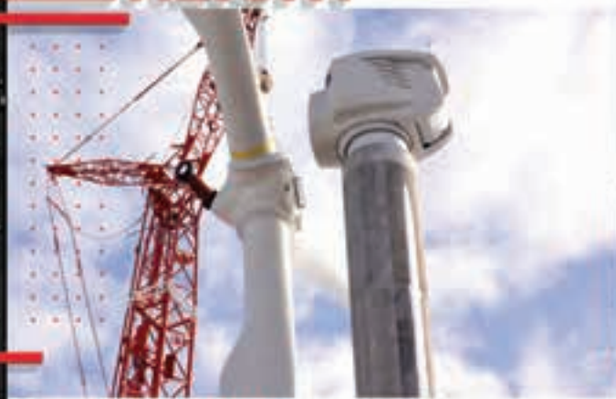
100 METER TALL (328 FEET) PRECAST WIND TURBINE TOWER
