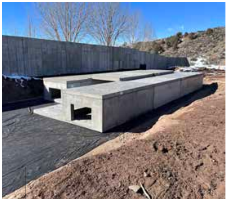
Oldcastle Infrastructure manufactured 13 modules, each of which was 4 feet high.
