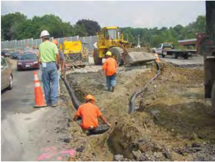
Figure 2-16. Installation of pavement drainage prior to the use of PCP panels.
