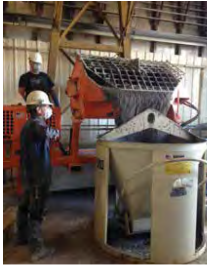
Figure 13-21. Mixed polymer concrete being discharged from a mixer into a concrete bucket.
