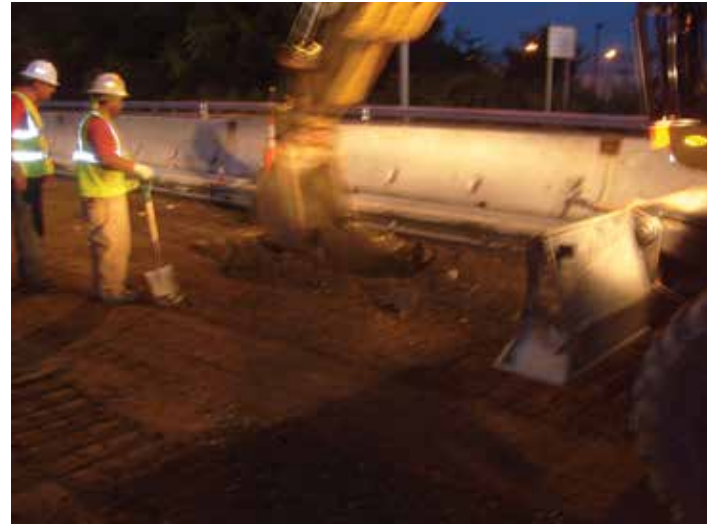
Figure 8-29. Spot repair during subbase preparation.
