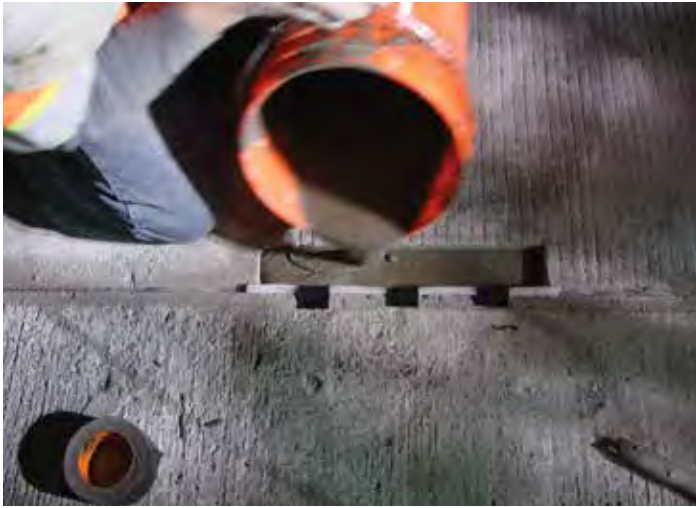
Figure 11-3. Two layers of foam (with black tape adhered to the near panel) were used along this transverse joint to retain the joint reservoir for the joint sealing material while repair material was installed.
