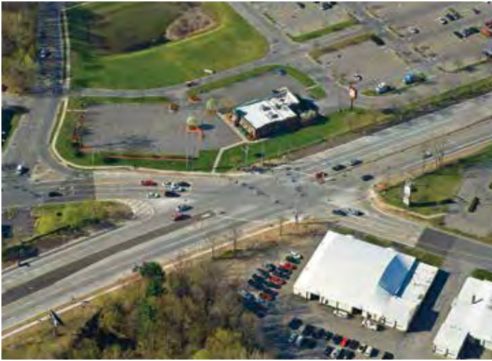
Figure 3-14. Aerial view of the intersection of Route 7 and Nott Street in Rotterdam, N.Y.
