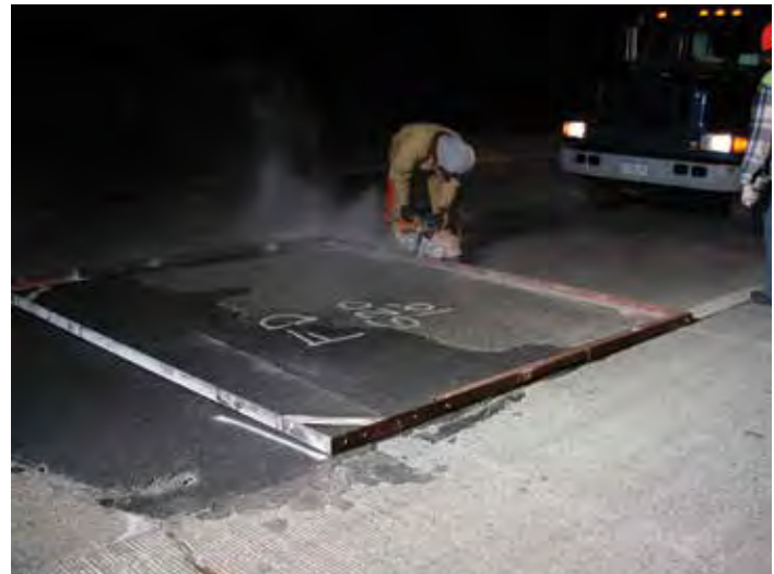
Figure 8-8. An example of a contractor-designed steel template being used to lay out and score saw cut lines for a single panel.
