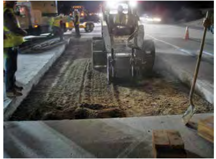
Figure 2-15. Removal of cement-treated base using a skid-steer-mounted milling machine on Interstate 210 in Tarzana, Calif.
