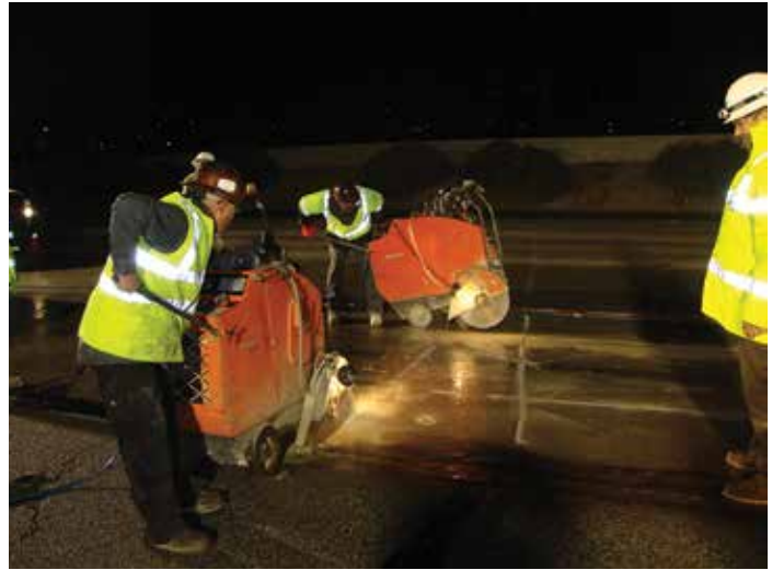
Figure 13-14. A transverse saw cut being made at the terminus of a single night’s installation. An additional saw making the longitudinal cut is seen in the background.
