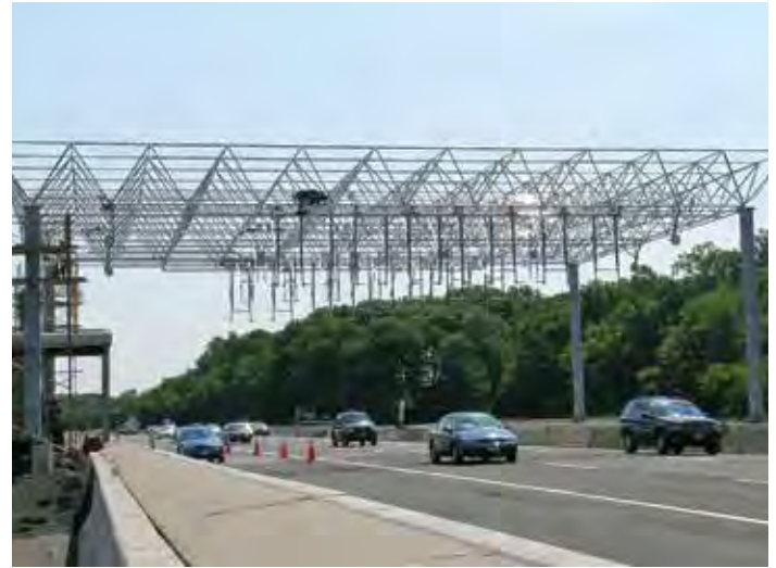
Figure 13-24. Overhead open-road-tolling equipment integrated with treadles embedded in precast panels below at New York Thruway Spring Valley toll plaza.
