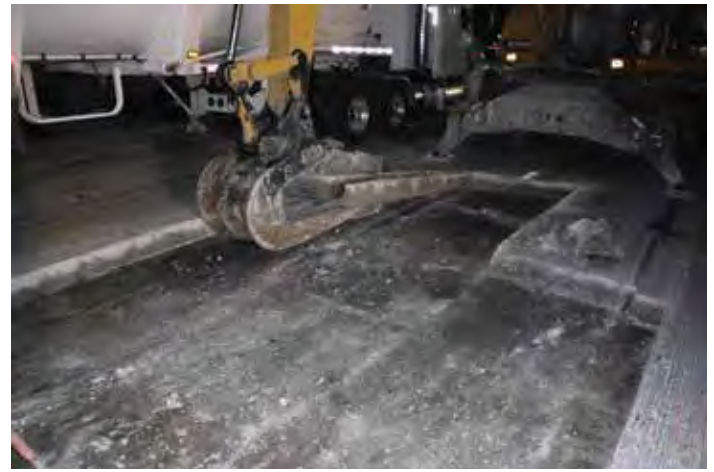
Figure 8-23. Removal of existing pavement using the excavator method with a slab-crab.
