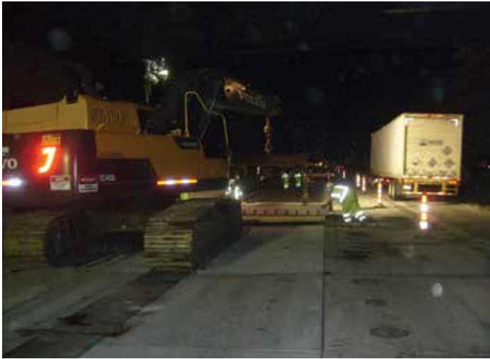
Figure 9-50. A track-mounted excavator placing a PCP panel under an overpass on Interstate 94 in Kalamazoo, Mich.
