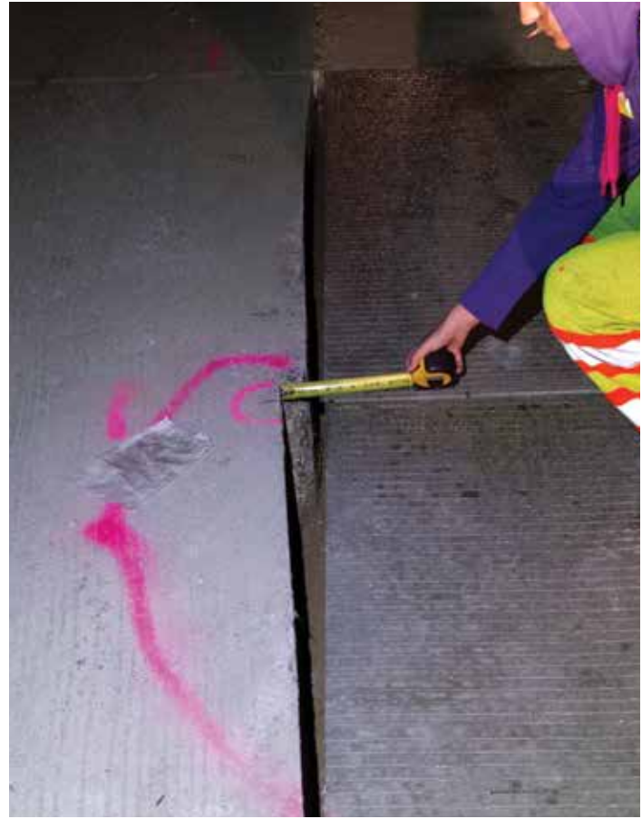
Figure 8-13. Example of an inaccurately sawed longitudinal joint.
