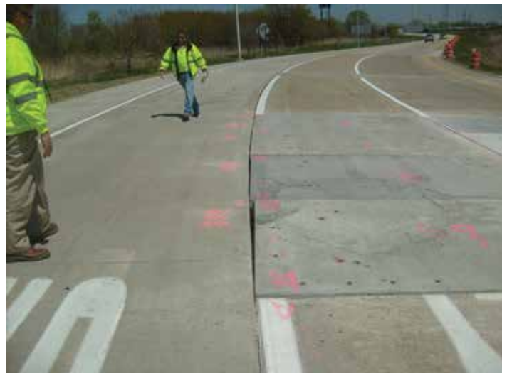
Figure 8-11. Example of a “saw-tooth” longitudinal joint created because the end cut, seen in the foreground, was not laid out and cut radially to the horizontal curve.
