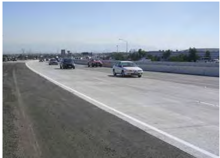
Figure 3-9. Lane replacement of a curved portion of Interstate 15 near Ontario, Calif., using JPrCP.
