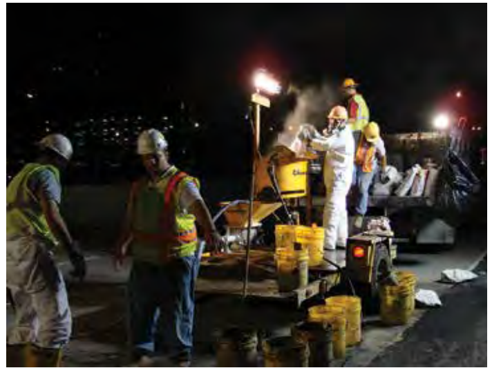
Figure 10-18. On-the-job training of a grout crew.
