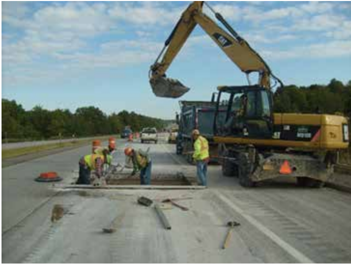
Figure 8-26. The versatile rubber-tire excavator can be used for removal, rough grading and placement of new panels up to 10 feet by 12 feet.
