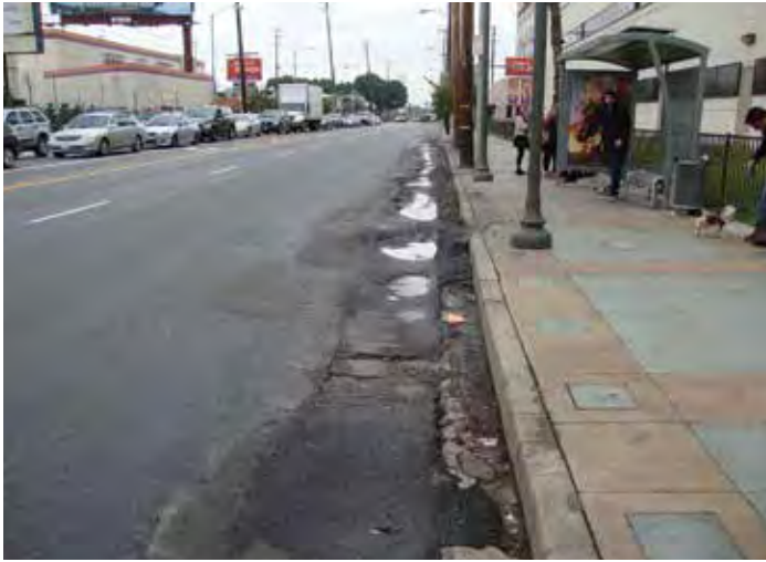
Figure 3-24. Bus pad pavement prior to replacement in North Hollywood, Calif.
