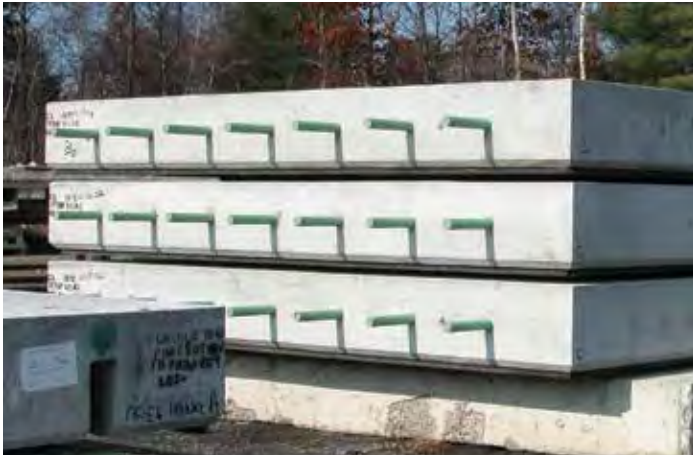
Figure 4-16. Half-embedded dowels in a JPrCP panel.
