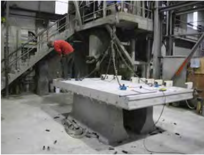
Figure 7-26. Panel placed on waist-high stands to facilitate stripping of slot formers, post-pour checking and panel detailing.
