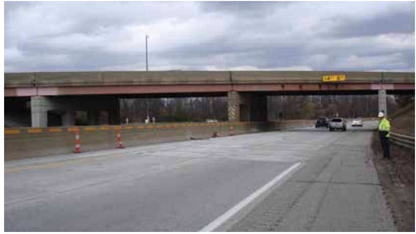
Figure 3-27. Completed repairs beneath an overpass on eastbound Interstate 94 (Business Loop) near Kalamazoo, Mich.
