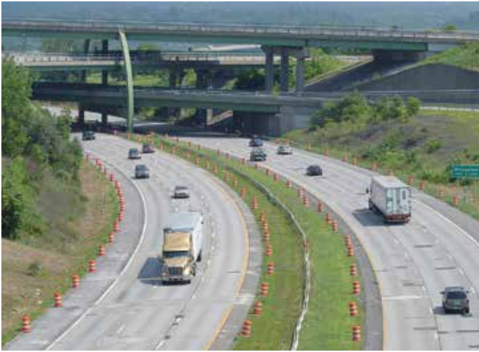
Figure 3-4. Use of precast panels for joint and mid-slab crack repairs in 62-foot-long slabs.
