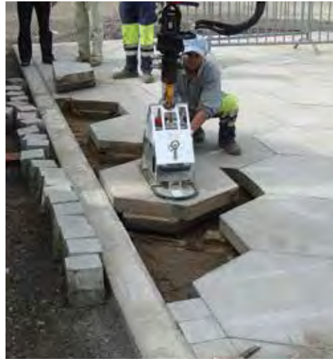
Figure 13-11. Hexagonal removable urban pavement system installed in Nantes, France.
