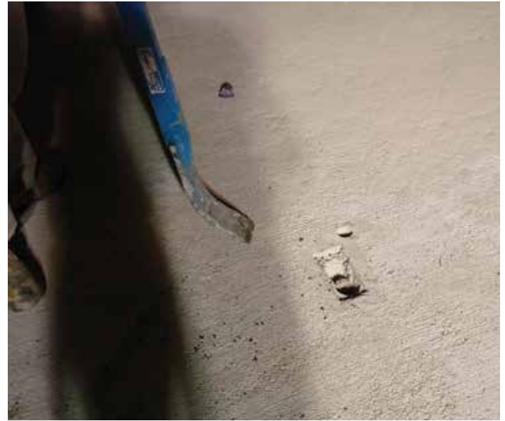
Figure 12-13. Recesses required for “dogbone” lifting pins are elliptical in shape, providing little resistance to grout pop-out.
