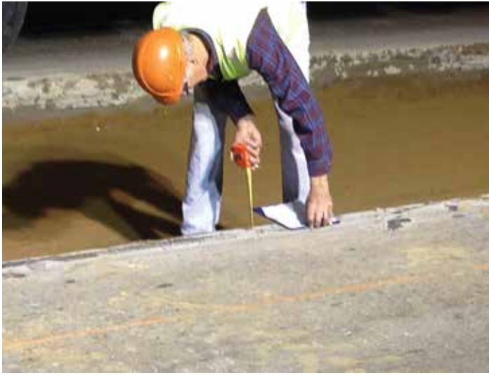
Figure 10-10. A DOT inspector checks the finished elevation and grading of the subbase.
