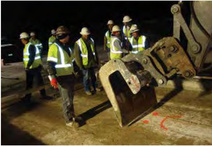
Figure 8-31. Trimming isolated high spots in CTB (red marks) with an excavator bucket.
