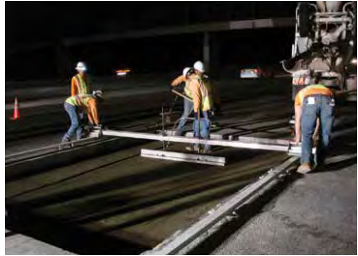
Figure 9-2. Workers use rails set to specific elevations to provide an accurate grade reference irrespective of the undulating existing pavement underneath.
