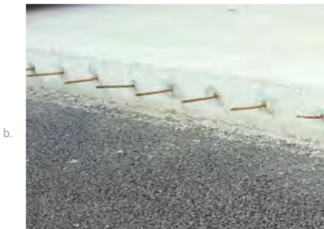
Figure 4-17. Schematic of a tied longitudinal construction joint with optional keyway and photo of tie bars along longitudinal joint. Sources: a. American Concrete Pavement Association; b. Pavement Engineering and Research Associates, LLC
