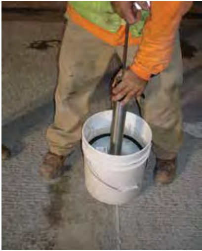
Figure 11-35. A standard caulking gun being charged with silicone sealant.
