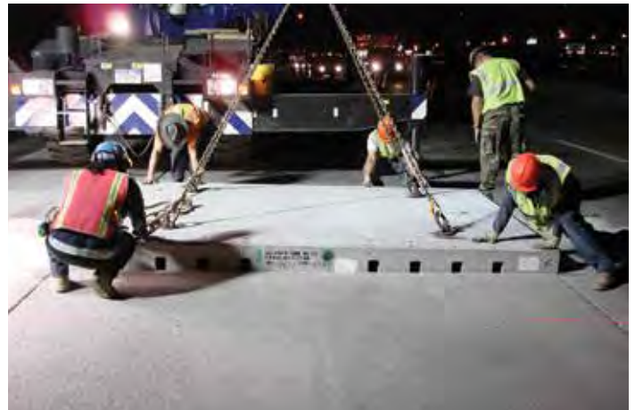
Figure 4-33. Panel being moved with four-point lift using lift inserts.
