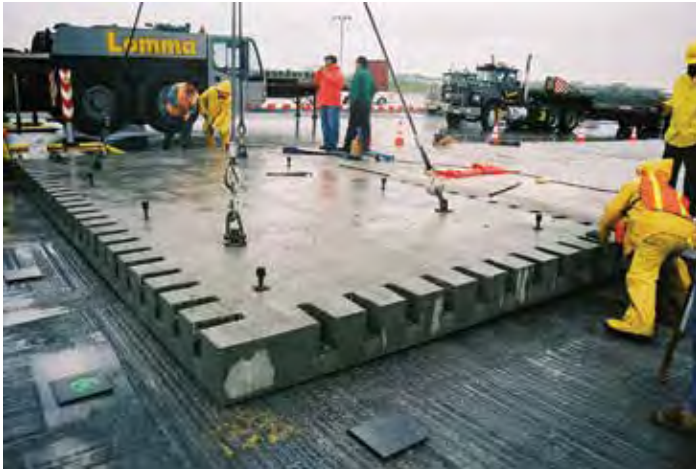
Figure 3-31. Installation of precast taxiway panels with leveling bolts at LaGuardia Airport.
