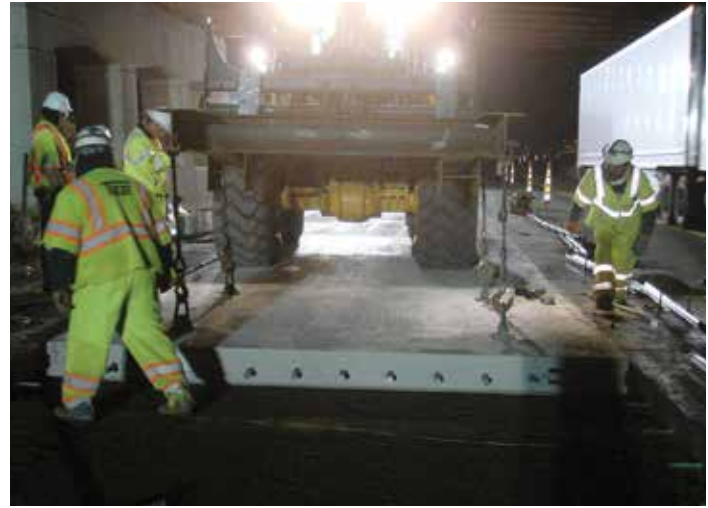
Figure 9-42. Installation of a bottom-slot precast panel over tie bars drilled in vertical faces of adjacent existing pavement.
