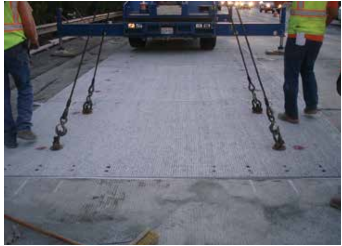
Figure 9-53. All the panels in the lane replacement repair area shown here were placed to leading end marks so the last panel being set precisely fits the space left by the previously placed transverse saw cut.
