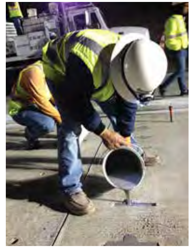
Figure 9-32. Latex grout being poured into the narrow top slot of the Barra Glide system.
