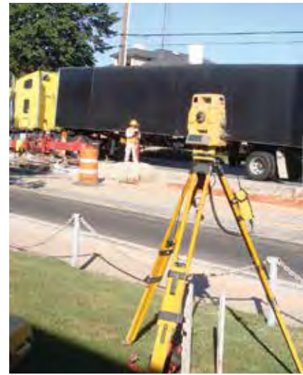
Figure 10-11. A surveyor uses a total station to establish panel points and grades for continuous PCP.
