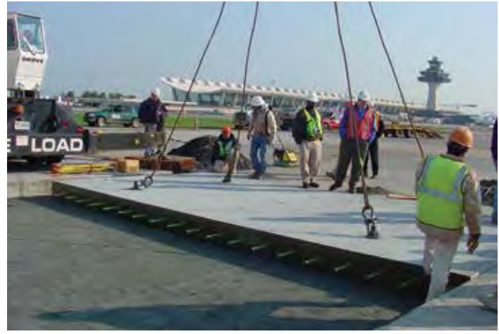
Figure 3-32. Installation of precast taxiway panels on precision-graded base at Dulles International Airport.
