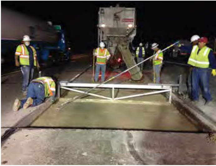
Figure 10-14. Two concrete finishers working behind four workers screeding newly placed lean concrete subbase.
