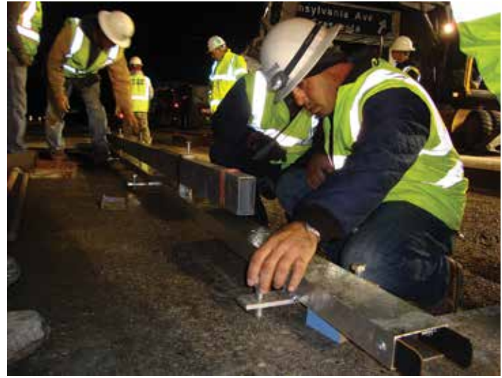
Figure 10-7. A grading crew checks and adjusts screed rails to ensure an accurate grading frame of reference.
