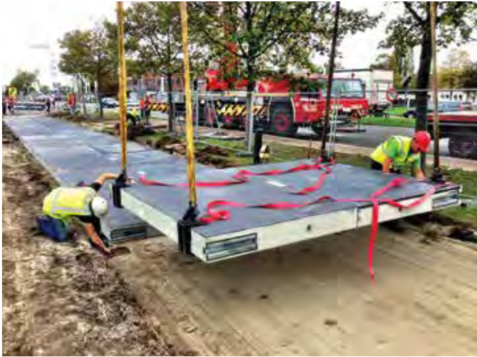
Figure 13-29. Precast power-generating panels being installed on accurately graded bedding material.
