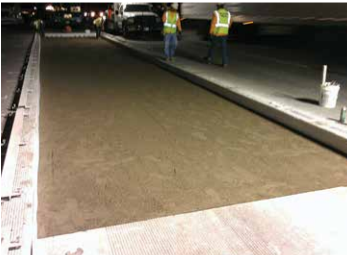
Figure 3-6. Long interior repair area prepared for installation of JPrCP panels.
