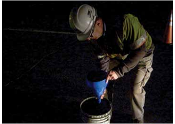
Figure 9-14. A worker performs a flow test in accordance with ASTM C939 to ensure proper consistency of the bedding grout.
