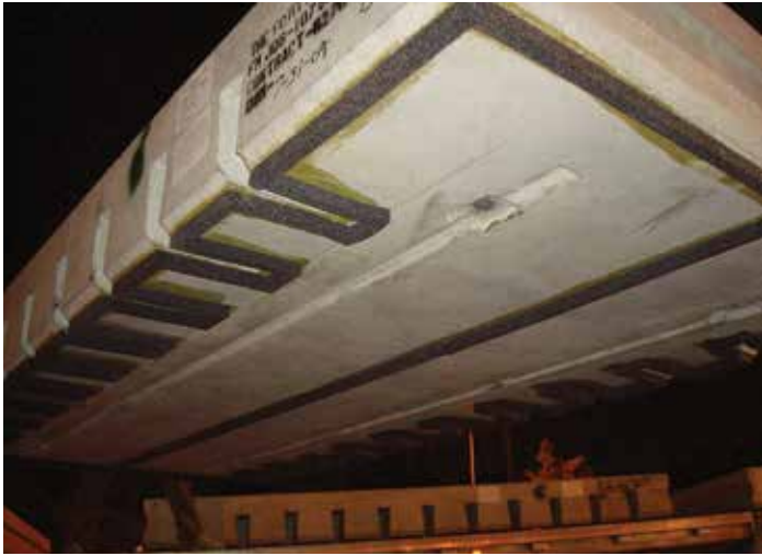
Figure 4-10. Grout distribution channels and gasket material on a Super-Slab JPrCP panel.
