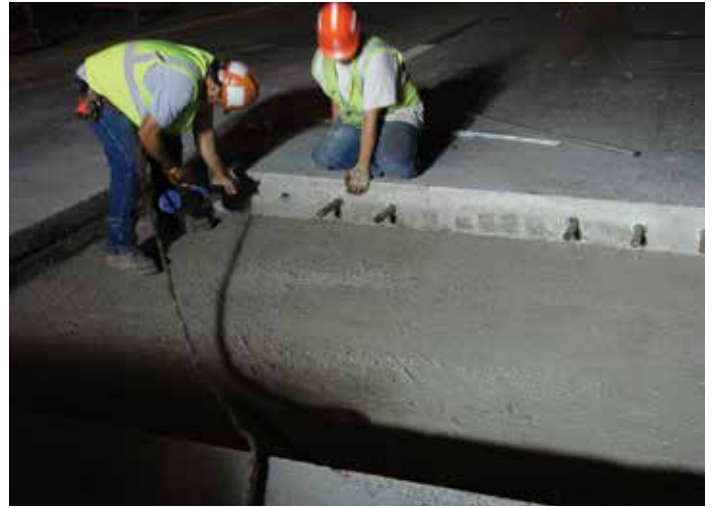
Figure 9-26. An air-powered, epoxy injection (caulking) gun is used to install anchoring epoxy. White epoxy retainer discs are visible around the dowels.
