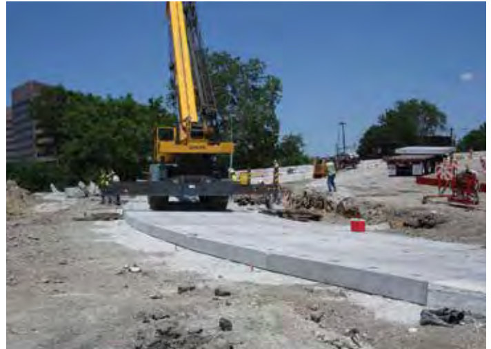
Figure 3-10. “Tight-radius” single-lane ramp in Chicago, Ill., that was replaced during a single weekend closure.
