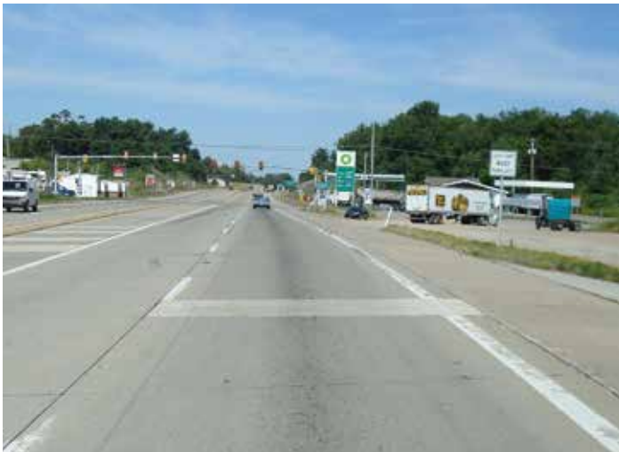
Figure 4-3. Concrete pavement with widened outside lane construction.
