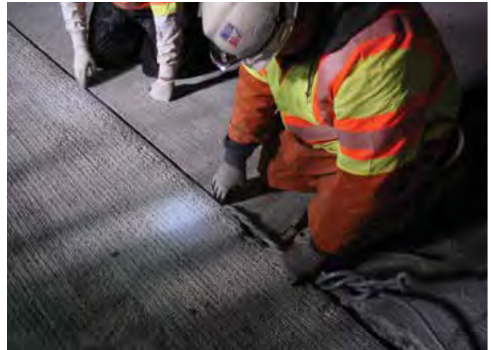
Figure 11-32. Small-diameter backer rod being braided together to fill a variable-width longitudinal joint prior to sealing.
