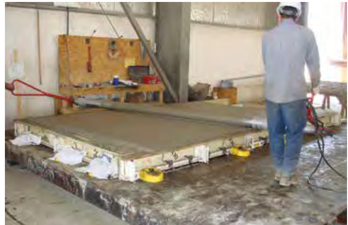
Figure 7-10. Magnetically anchored side rails being used on all four sides of a single-panel form.
