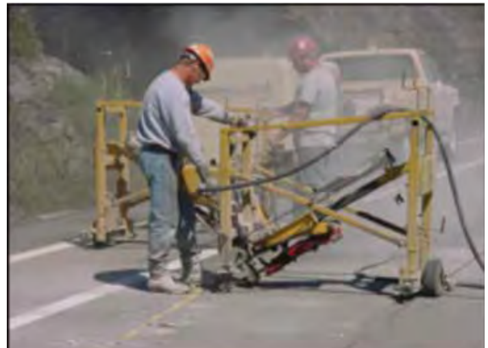
Figure 9-40. A worker uses a pneumatic drill to create cross-stitch holes across a longitudinal slab crack.
