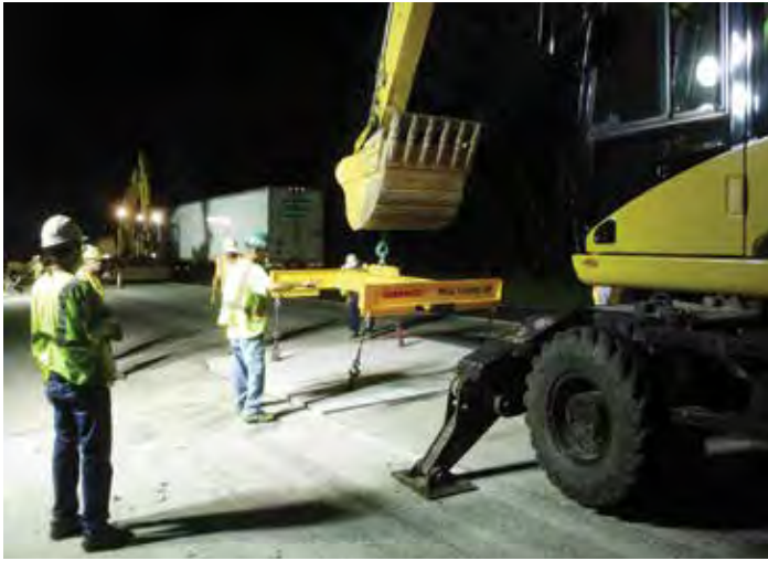
Figure 9-47. The outrigger of this rubber-tired excavator is located outside of the PCP panel area.
