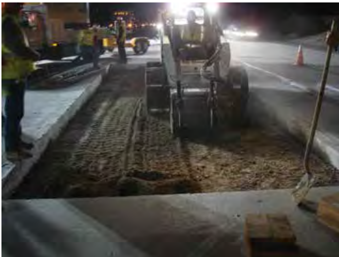
Figure 8-32. A skid-steer-mounted milling head trimming a large area of CTB.
