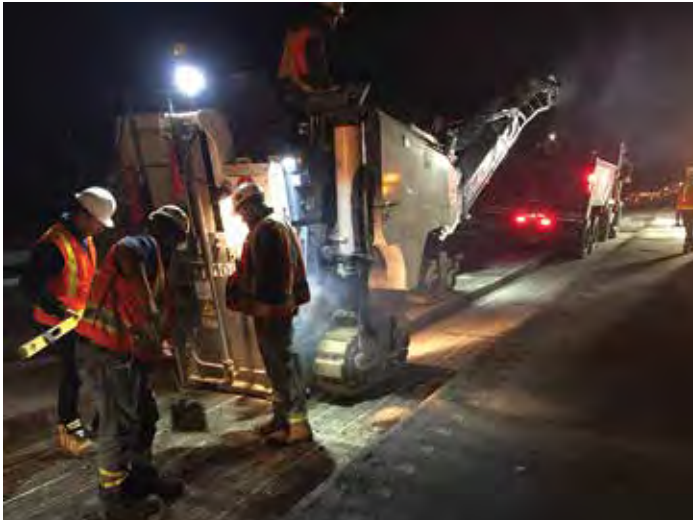
Figure 13-15. A 1.2-meter-wide milling machine makes a full-depth pass.
