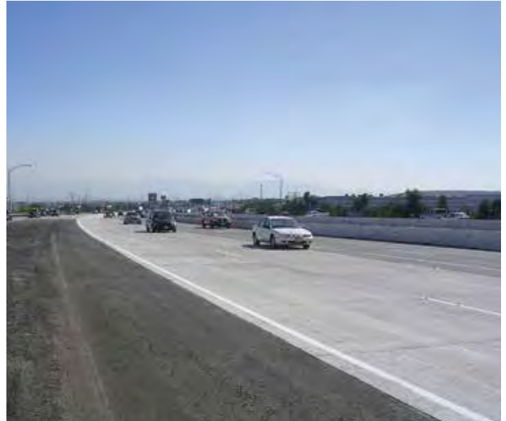
Figure 12-1. Interstate 15 in Ontario, Calif., carries approximately 200,000 vehicles per day and includes high-quality precast panels (seen in the left two lanes) that were installed in a series of eight-hour night work windows.
