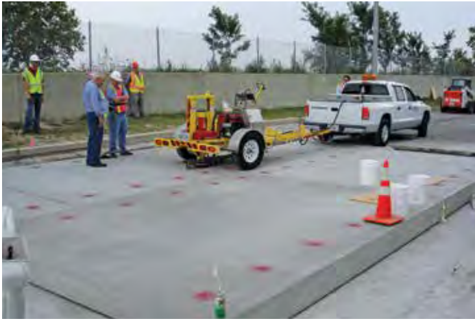
Figure 10-2. Falling weight deflectometer equipment measuring load transfer efficiency at a trial installation in Chicago, Ill.
