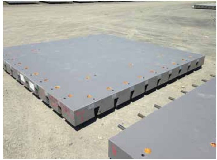
Figure 13-22. Finished panels stored at the precast yard prior to shipment to the job site.
