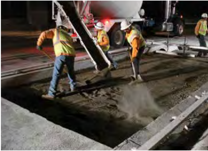
Figure 9-5. Cement-treated bedding material being discharged from a standard concrete truck.
