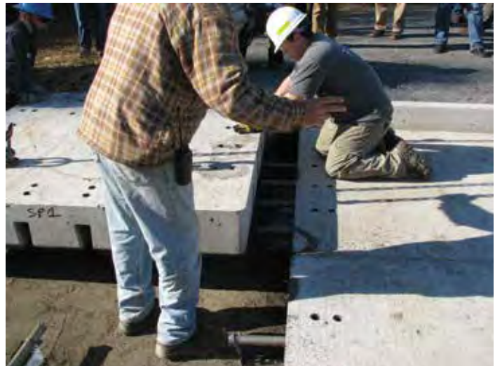
Figure 13-12. Super-Paver unit being installed over Super-Dowels in adjacent units.
