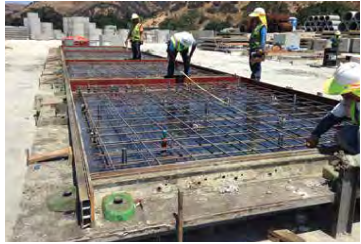
Figure 7-15. QC check of panel lengths just prior to concrete placement.
