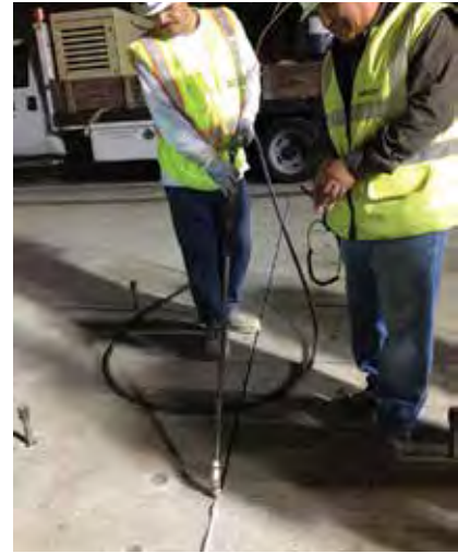
Figure 11-36. Silicone sealant being applied through a nozzle attached to a pressurized drum.
