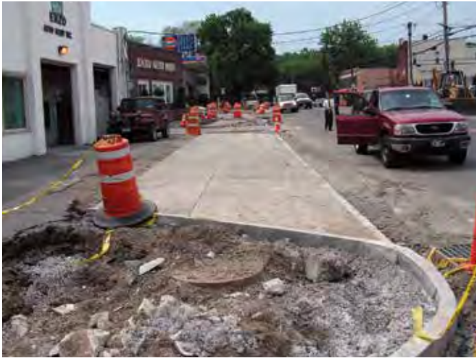
Figure 13-20. Non-planar, specially shaped precast panels were manufactured to meet the adjacent granite curb and pronounced surface contours while providing continuous commercial access.
