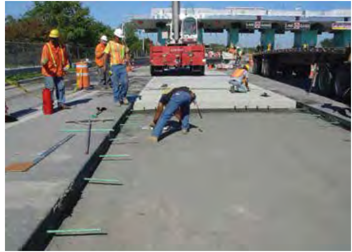
Figure 9-48. Both sets of outriggers on this hydraulic crane are positioned on existing pavement.
