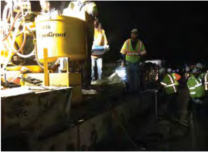
Figure 9-19. A dual-drum, high-capacity mixer/pump mounted on a service trailer with an adequate supply of grout and water and a safe working space.
