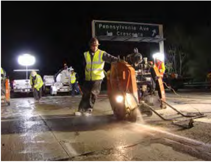
Figure 10-12. A sawing crew consisting of two saw operators and one slurry cleanup man.
