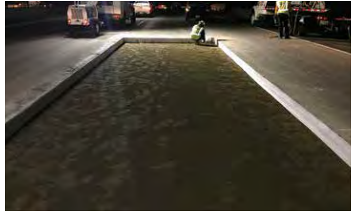
Figure 11-29. 1/2-inch-thick white isolation foam attached to the longitudinal edge of the existing pavement.
