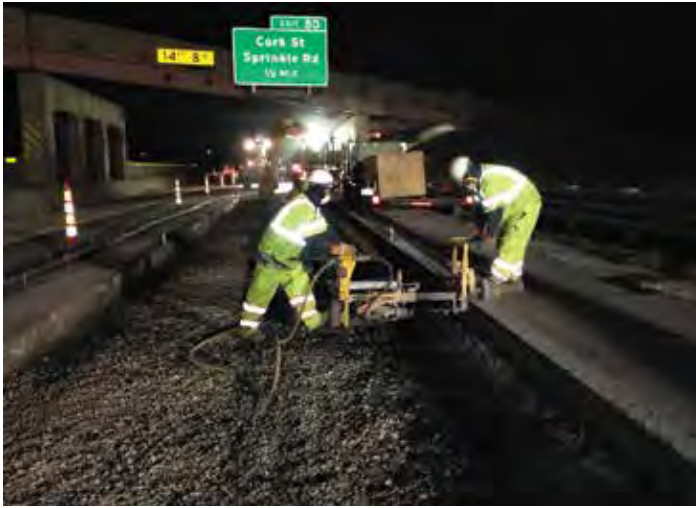
Figure 9-41. A single-bit air drill used for drilling tie bar holes at correct locations.
