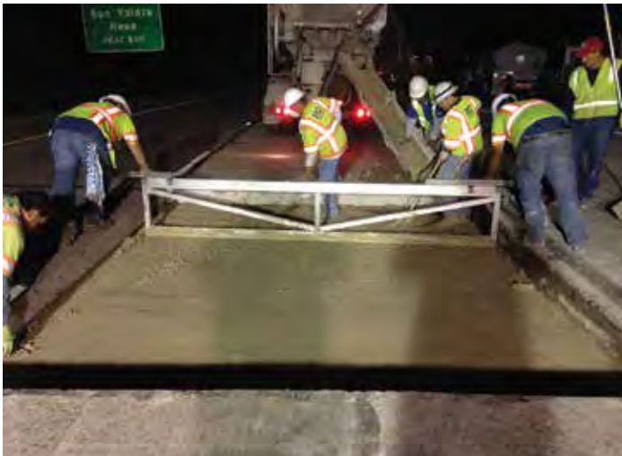
Figure 9-7. A wheel-mounted concrete screed using a pre-set rail on one side of the hole and the existing pavement on the other as a grade reference.
