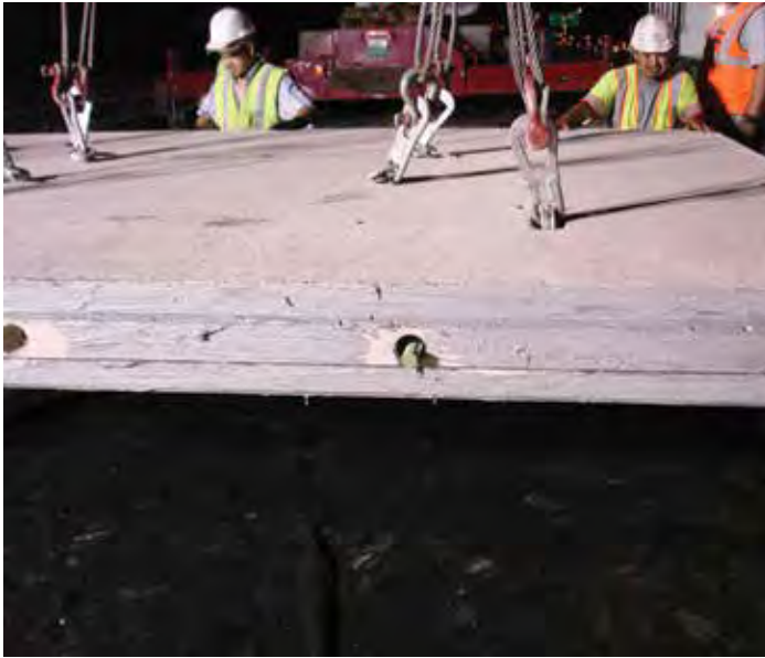
Figure 12-12. “Dogbone” lifting pins are favored by some precasters because they allow quick and safe attachment of lifting cables to precast panels.
