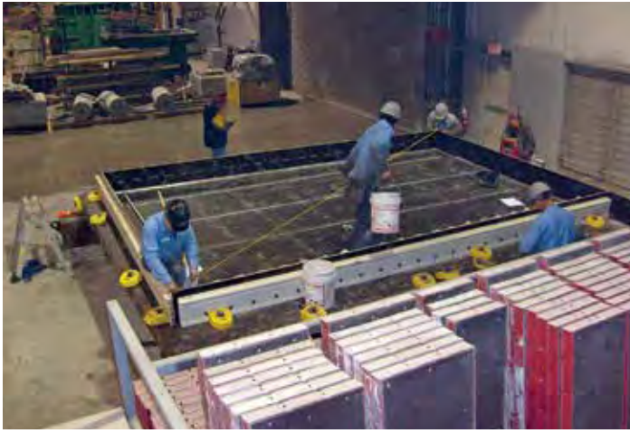
Figure 7-14. Checking form diagonals during form setup.
