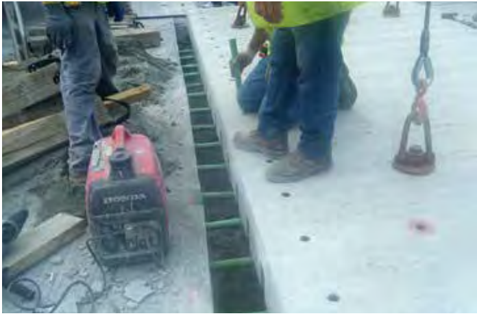
Figure 11-11. The over-width transverse joint in this photo resulted from incorrect saw cut layout in the existing pavement on the left. The error was not discovered until the precast panel on the right was placed.
