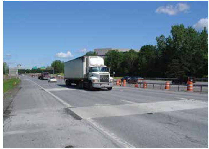
Figure 3-3. Six-foot-long, full lane-width joint repair panels in adjacent lanes.
