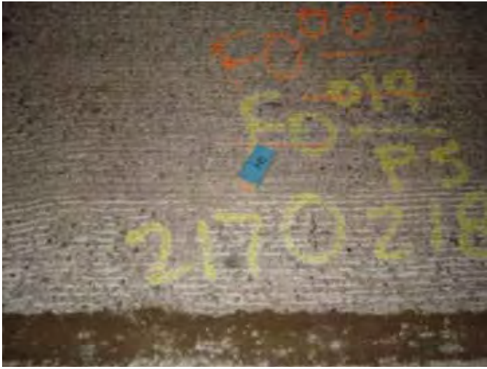
Figure 8-12. Example leading end mark for a panel designated number 217 (see black line perpendicular to pavement edge in yellow circle).
