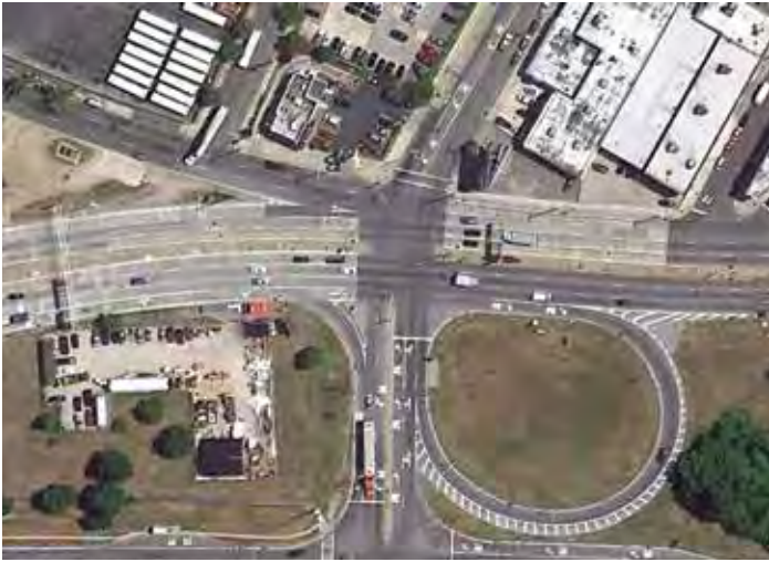
Figure 3-16. Aerial view of the Rockaway Boulevard-Farmers Boulevard intersection in Queens, N.Y.
