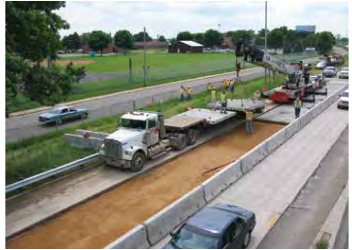
Figure 9-46. A 65-ton capacity hydraulic crane picking panels from a truck positioned in front of, rather than alongside, the crane.
