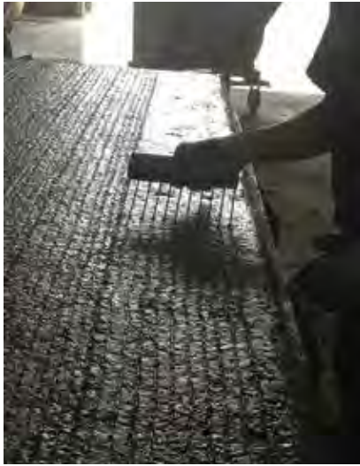
Figure 7-24. Use of a narrow, custom-width rake to texture a narrow strip at the edge of a panel.
