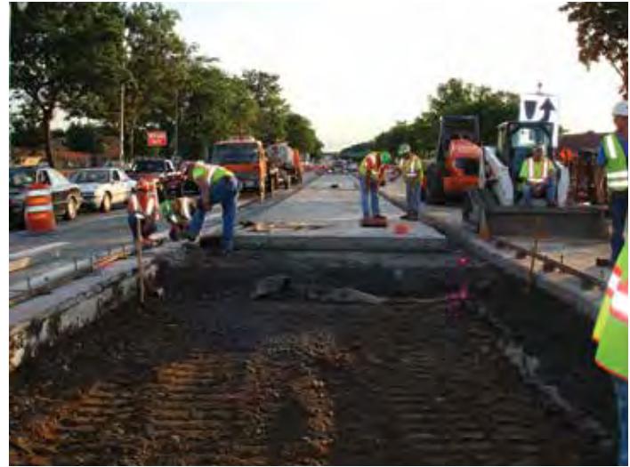
Figure 8-27. An example of undercutting 1 foot prior to replacement with geo-fabric, new subbase material and JPrCP panels.
