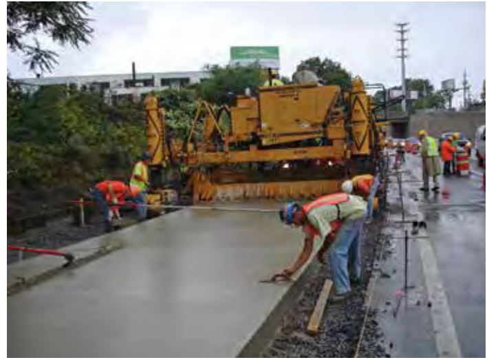
Figure 1-4. Plastic concrete extruded to correct grade and cross-slope behind slip-form paver.
