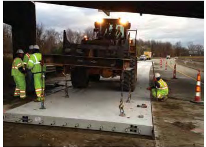
Figure 9-51. A large loader carrying and placing a PCP panel under an interstate overpass.
