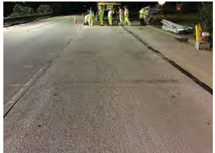
Figure 3-7. Example use of multiple JPrCP panels in a single repair.
