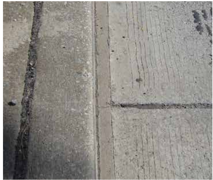
Figure 12-7. This 1.5-inch-wide, grout-filled longitudinal joint, located between an existing curb on the left and precast panels on the right, is performing well after being in service for more than five years.
