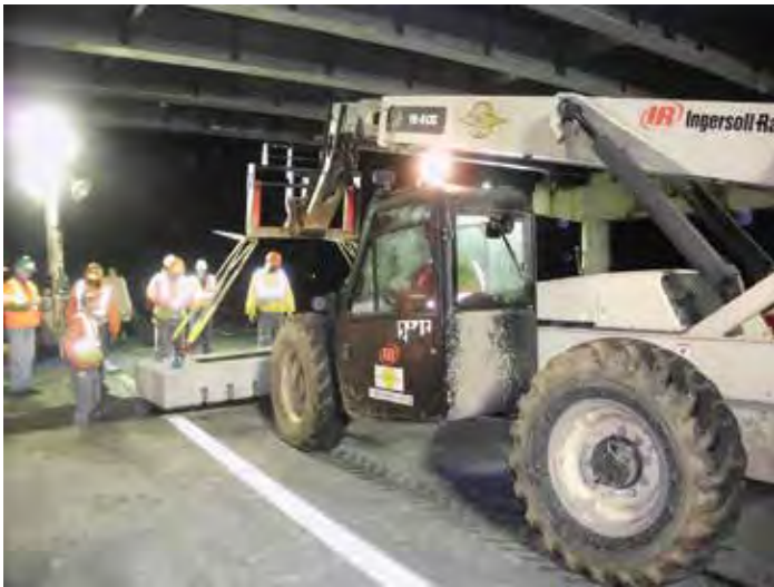
Figure 2-6. Example use of a fork truck to install PCP panels beneath an overpass.
