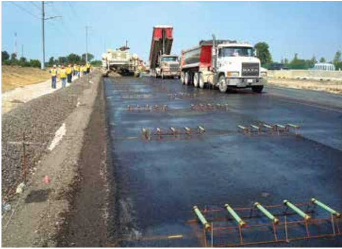
Figure 4-22. 2013 photos of conventional paving (left) and precast repairs (right) using only wheel path dowels on Illinois Tollway projects.
