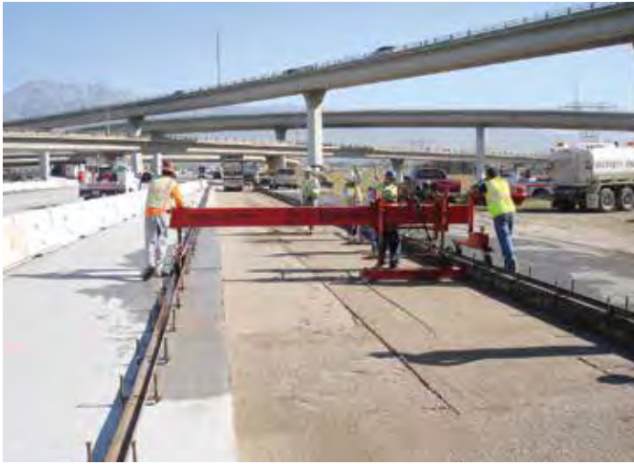
Figure 9-3. A larger, hand-operated grader controlled by pre-set grade rails set to specific elevations.
