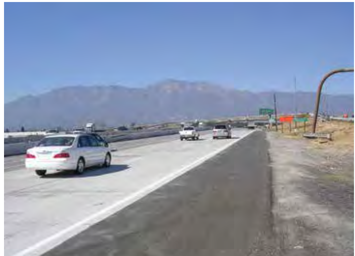
Figure 3-8. Tangent lane replacement of a portion of Interstate 15 near Ontario, Calif., using JPrCP.
