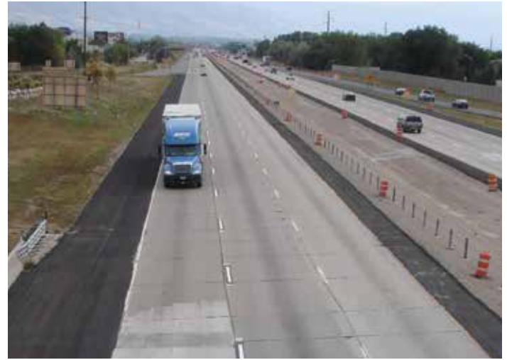
Figure 11-24. The existing pavement in the lower left corner of this photo was ground on both the approach and leave ends of a panel because the precast panel was placed too low.
