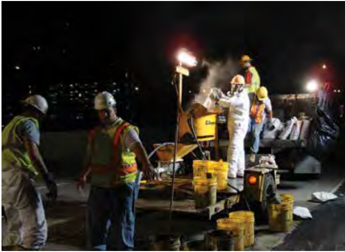
Figure 9-15. A grouting crew using a trailer-mounted batch-type mixer/pump.
