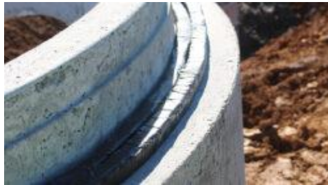
Apply Sealant Per Manufacturer's Recommendation
