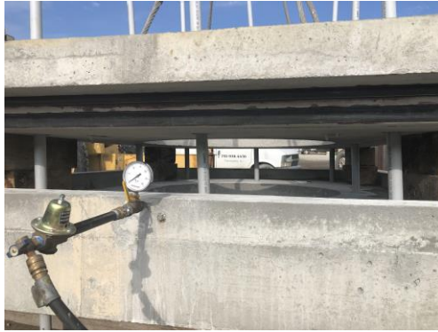
Photo credit Garden State Precast
