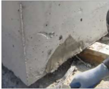
OVER FILL REPAIR AREA
