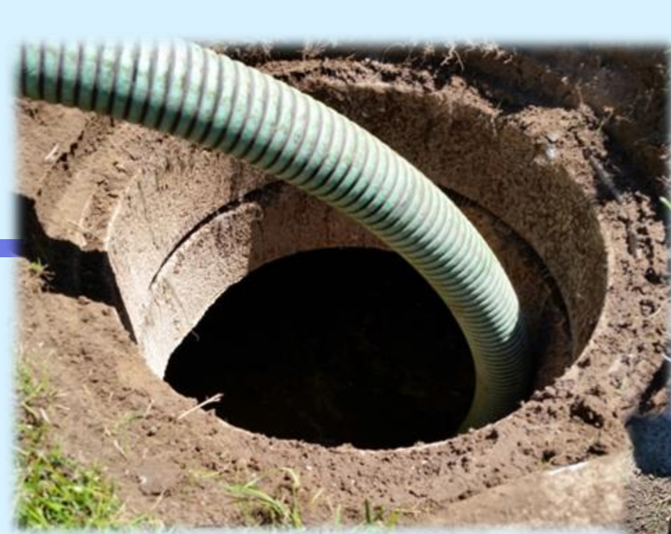
Septic Tank Inlet Riser
