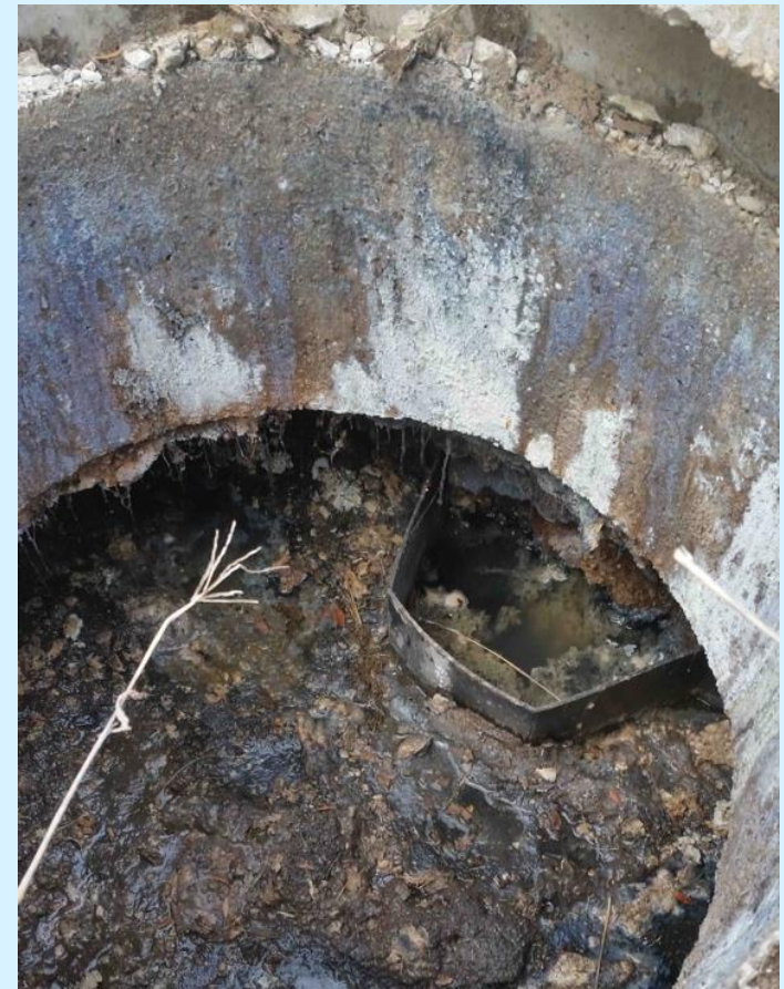
Open outlet baffles
