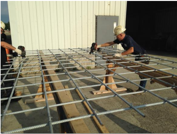
Tied Reinforcing Steel (rebar)
