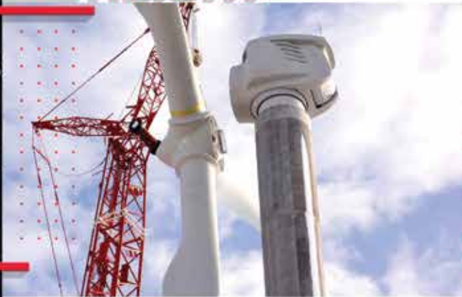
100 METER TALL (328 FEET) PRECAST WIND TURBINE TOWER
