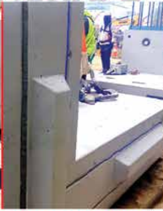
PRECAST & CAST-IN-PLACE COMBO BUILDING ACCESS TUNNEL
