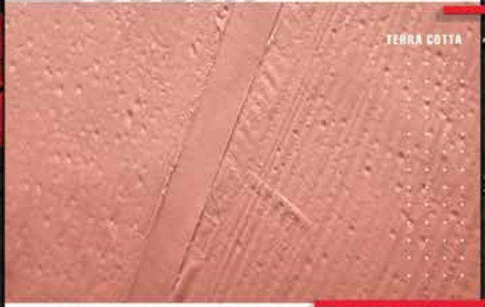
COLOR MATCHED WATERPROOF COATING & ELASTOMERIC JOINT SEALANT APPLIED TO ARCHITECTURAL CONCRETE JOINT
