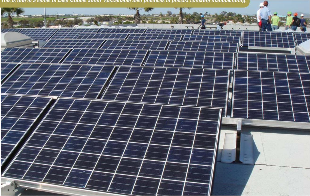
Solar panels supply electricity and occasionally enable to plant to send power back to the California energy grid.
