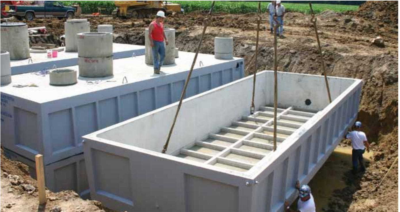
Baffles or tees are permitted to be precast monolithically with the tank. If baffles, tees or outlet filters are added, they shall be made of non-corrosive materials and be permanently connected with non-corrosive fasteners to either the inside of the tank or the outlet pipe.
