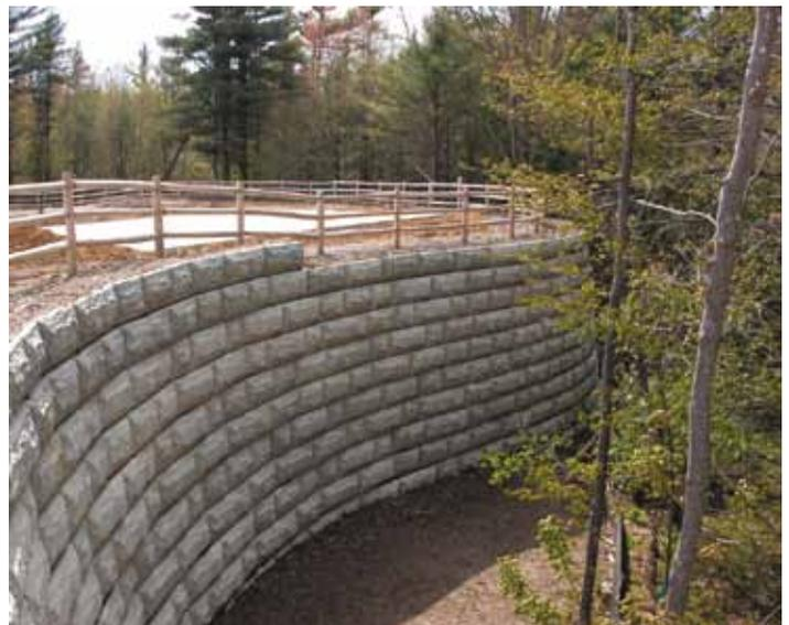
execution/installation. One "material characteristic" that can be of particular importance to retaining walls is the "product height tolerance" of the wall unit. Each manufacturer will have its own recommendation regarding acceptable plus or minus maximum height tolerance. In general, height dimensions should not vary more than a maximum of  $\pm 1/8$  inch (3 mm) for every 4 feet (122 cm) of the unit.
