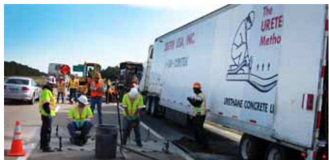
Figure 9: Urethane installation for the Roman Road system.
