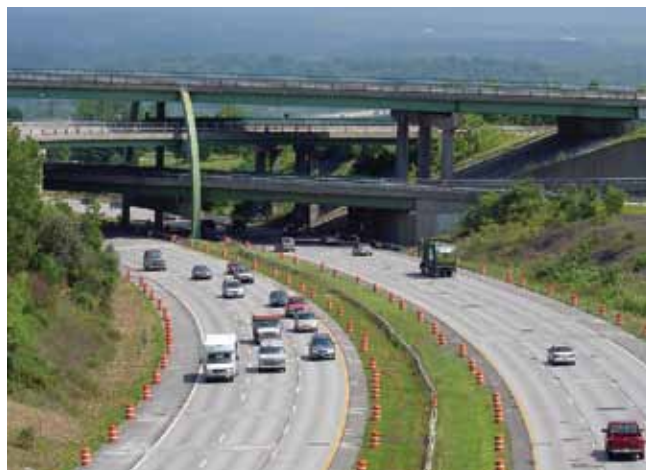
Figure 4: JPrCP installed intermittently in horizontal curves.
