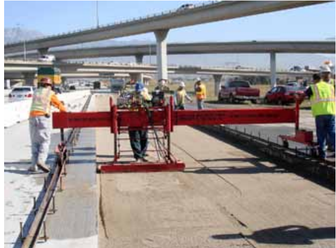
Figure 7: Precision grading for the Super-Slab® System.
