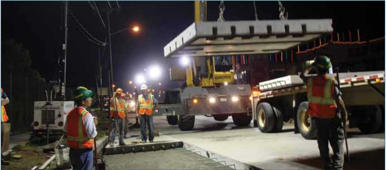
Figure 5: JPrCP installed in a pavement widening during overnight work windows.
