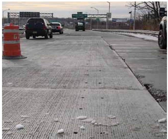
Figure 2: Precast slabs installed in frigid conditions – see ice in foreground.
