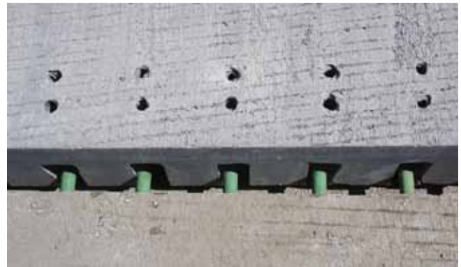
Figure 12: Installation of bottom slot Super Slab® system.
