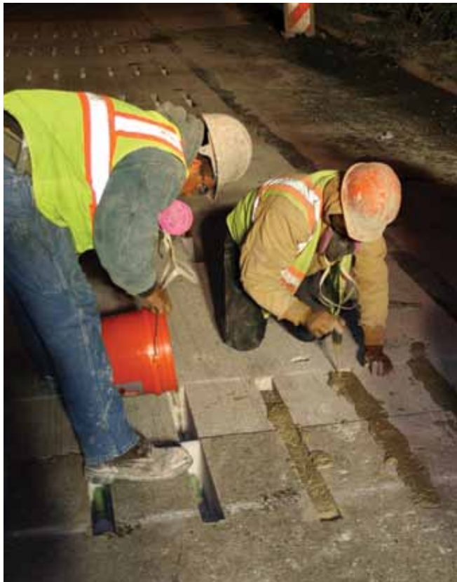
Figure 3; Fast-setting grout is installed over dowels positioned in dowel slots.
